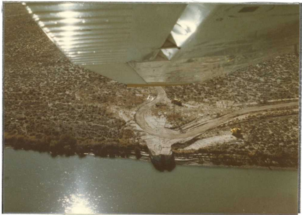
Aerial view of Johnson bulkhead, constructed by force account.
