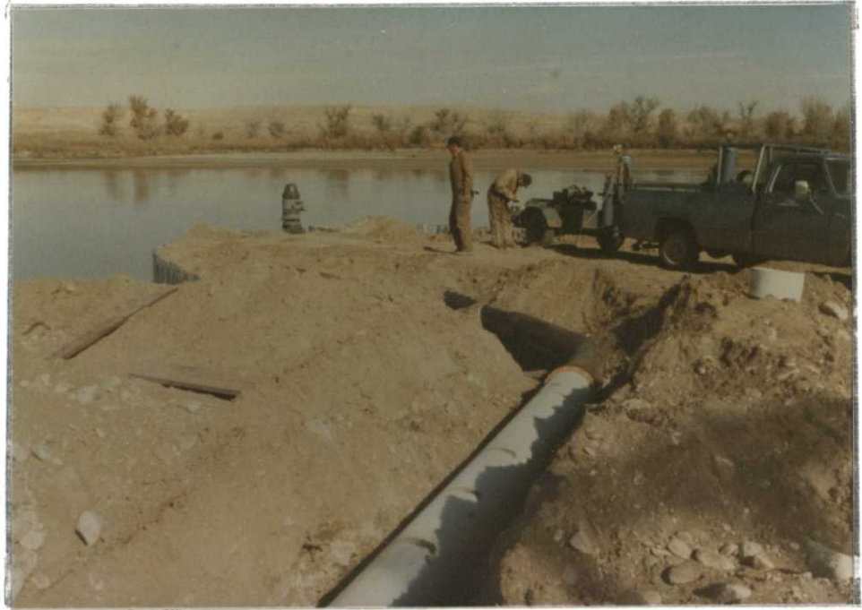
Littleton and Tornow completing installation of Johnson Bottom pump.
