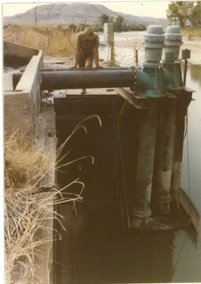
Littleton and two Leota pumps we installed.
