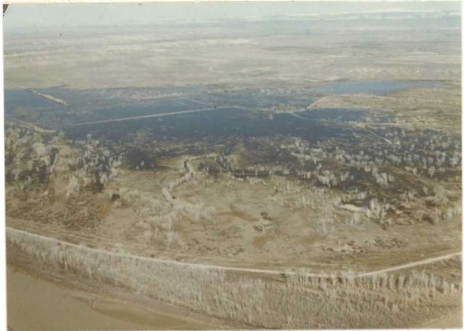
Aerial view of flooded Sheppard Bottom from the southeast, April 6, 1979.
