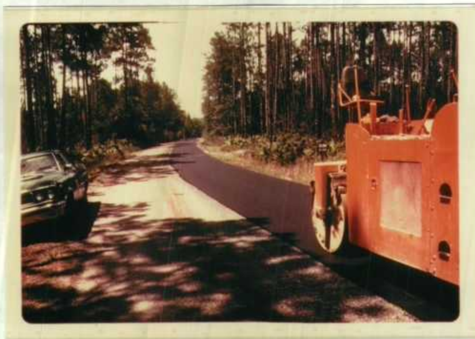
Resurfacing the Swamp Island Drive NS-16-77, Staff.
