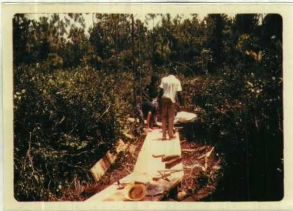
Y.C.C. constructed boardwalk -- "The Songbird Trail" NS-90-77, Staff.
