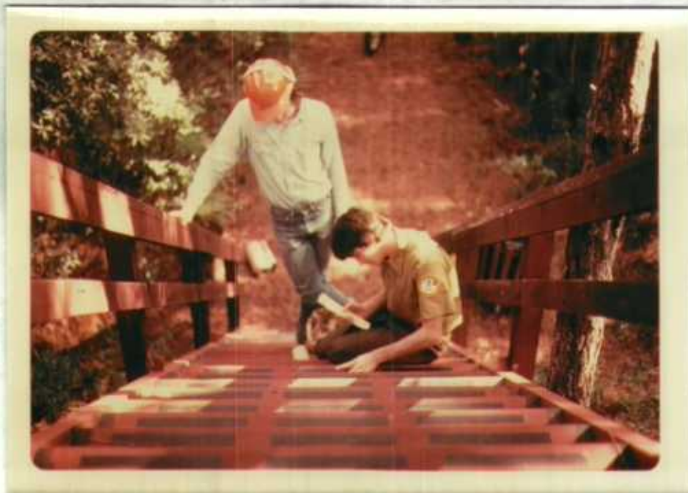
Applying non-skid material to tower steps. NS-94-77, Staff.
