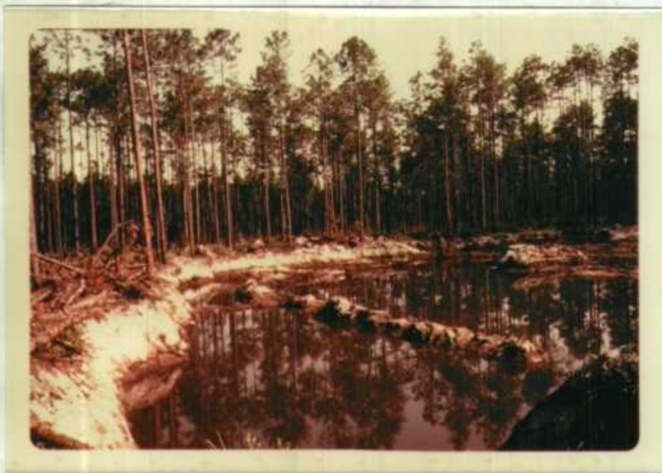
This Borrow Pit was the fill source for reconstructing the Swamp Island Drive. NS-18-77, Staff.
