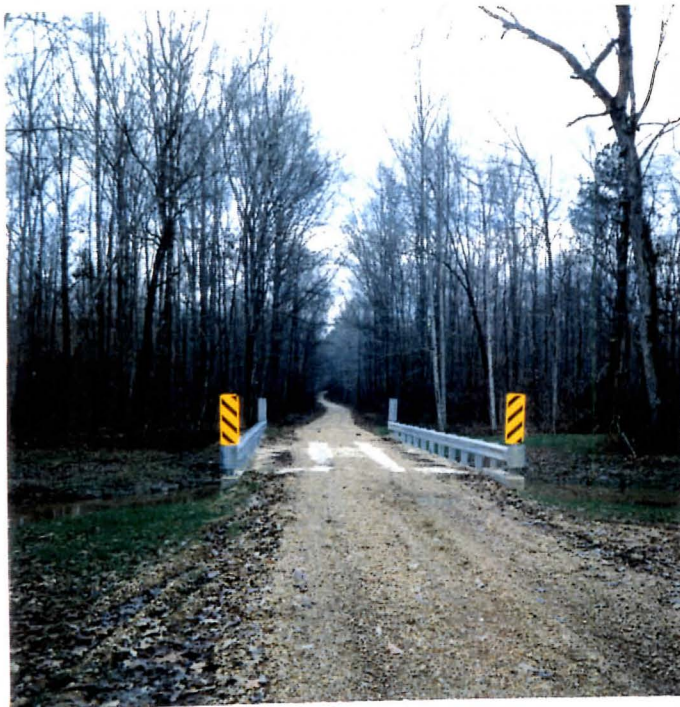
Same location, but the new bridge doesn't rattle. (17-96 Hall)
