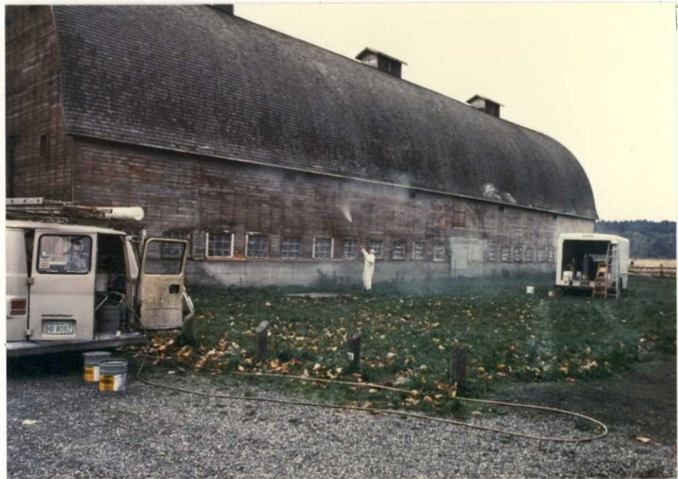
Figure 33. Pressure washing cleaned up the Barns before a clear sealant was applied to the outer surface.
