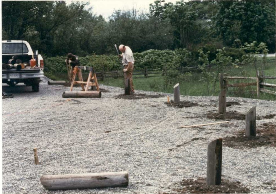
Figure 32. The finishing touches.
