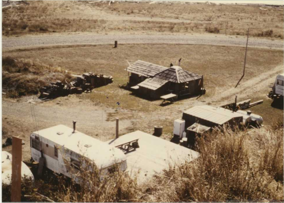
Figure 15. A classic example of hodge-podge development. This or these are not habitable structures and will be removed. 85-WBH
