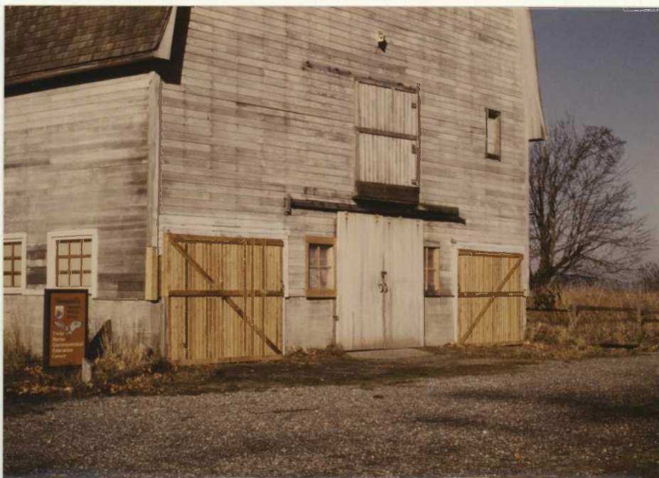
Figure 39. New doors on the twin barns. 85-SE
