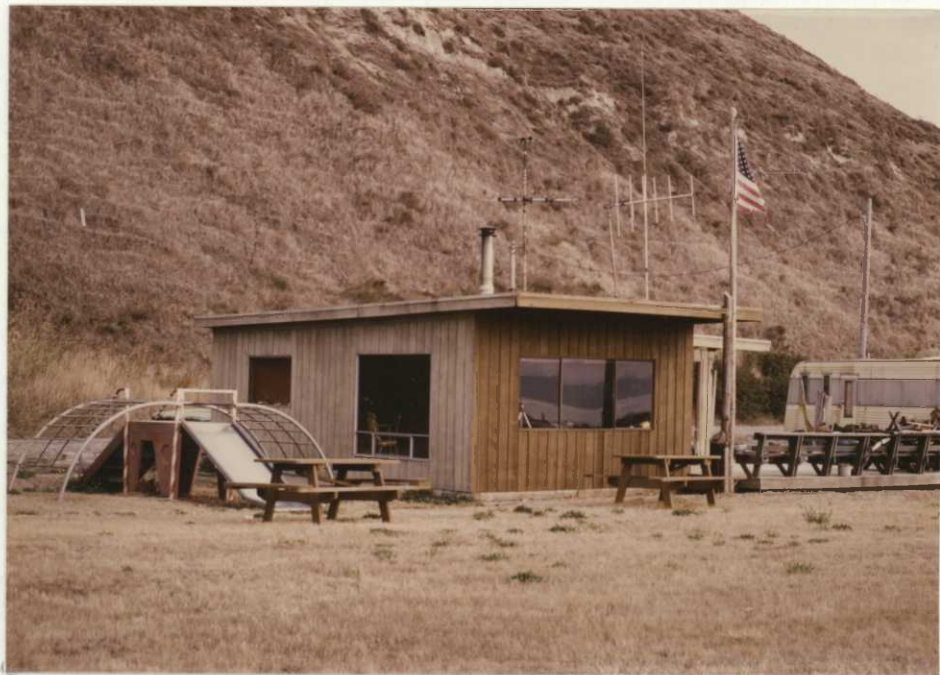
Figure 16. This habitable structure owned by Sound Properties, Inc. will become the on-site office for FWS personnel or volunteers. There will probably be no time to play. 85-WBH
