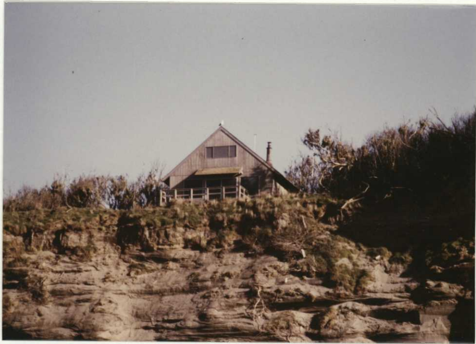
Figure 8. The habitable structure which will be occupied by volunteers. 85-WBH
