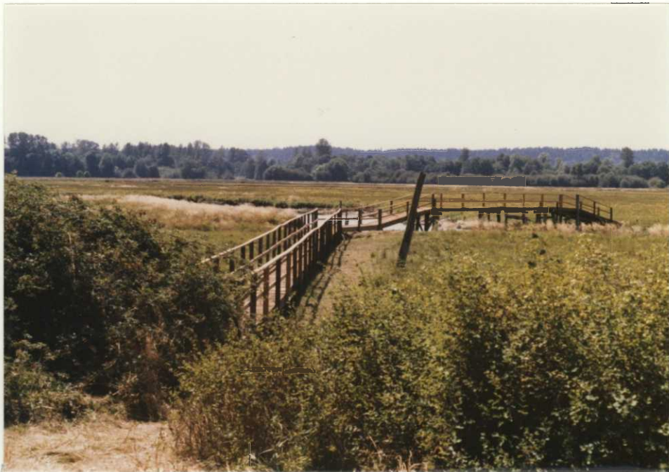
Figure 9. YCC's did a fine job constructing new boardwalk. 85-RW
