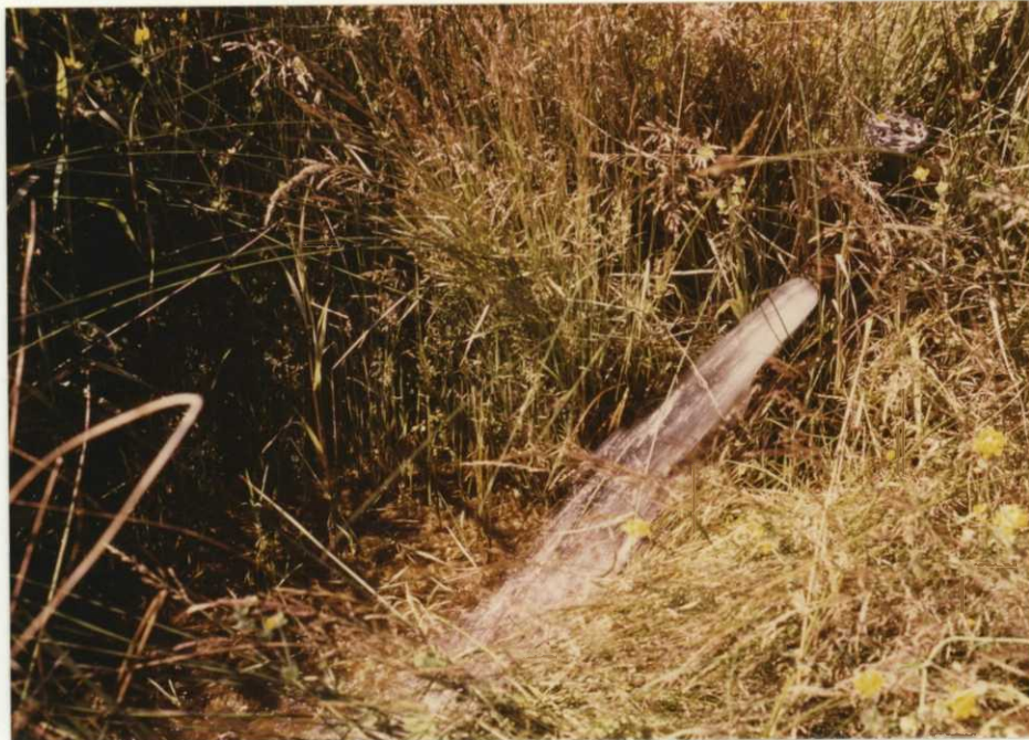
Figure 16. The six-inch Shannon Slough well provides adequate flow for water level maintenance. 85-SPT
