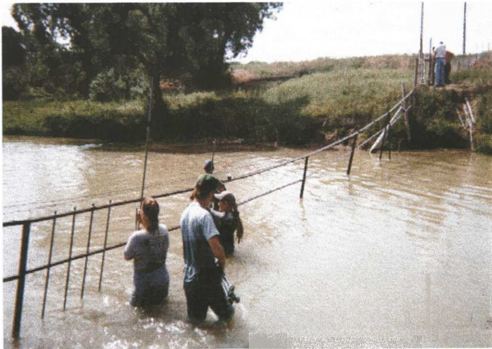
Figure 2. YCC designed and constructed a boundary "fence" across the fluctuating Lake Alice outlet that will permit debris to flow downstream yet keep cattle out.
