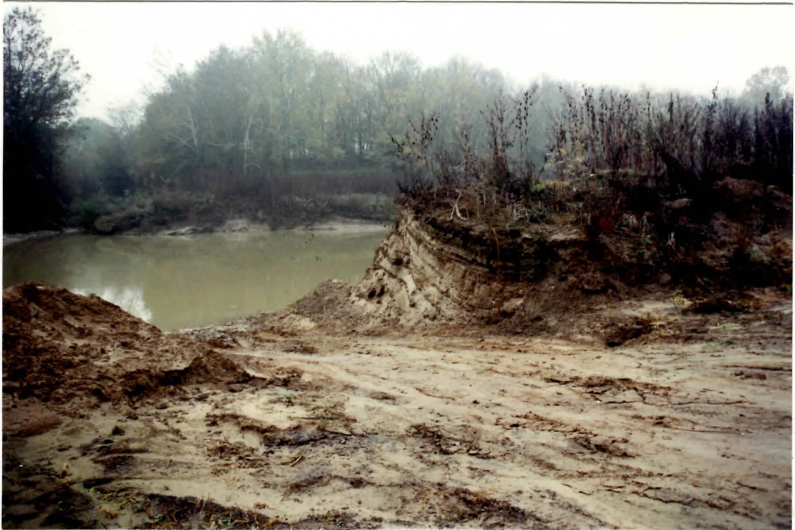
Easement violation (earth removal) on Prissock tract. LWD 97-7; 11/97; AH
