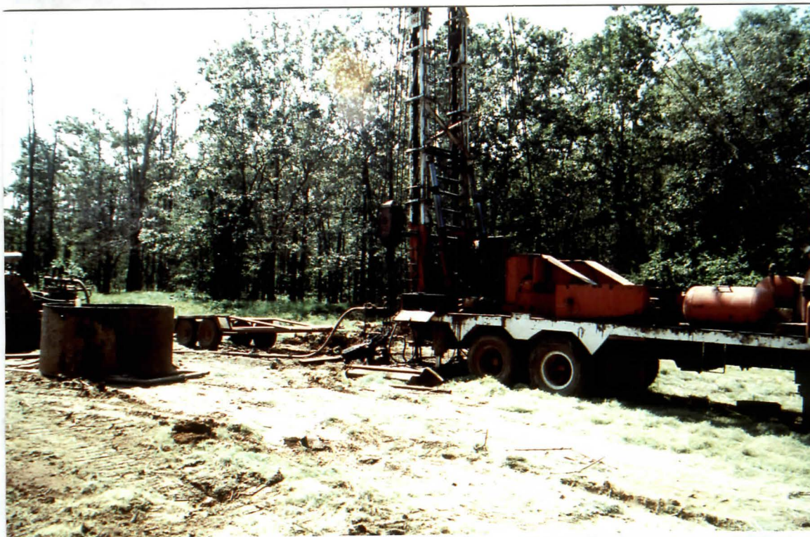
Plugging abandoned gas wells; DRB-97-3; 8/97; MS
