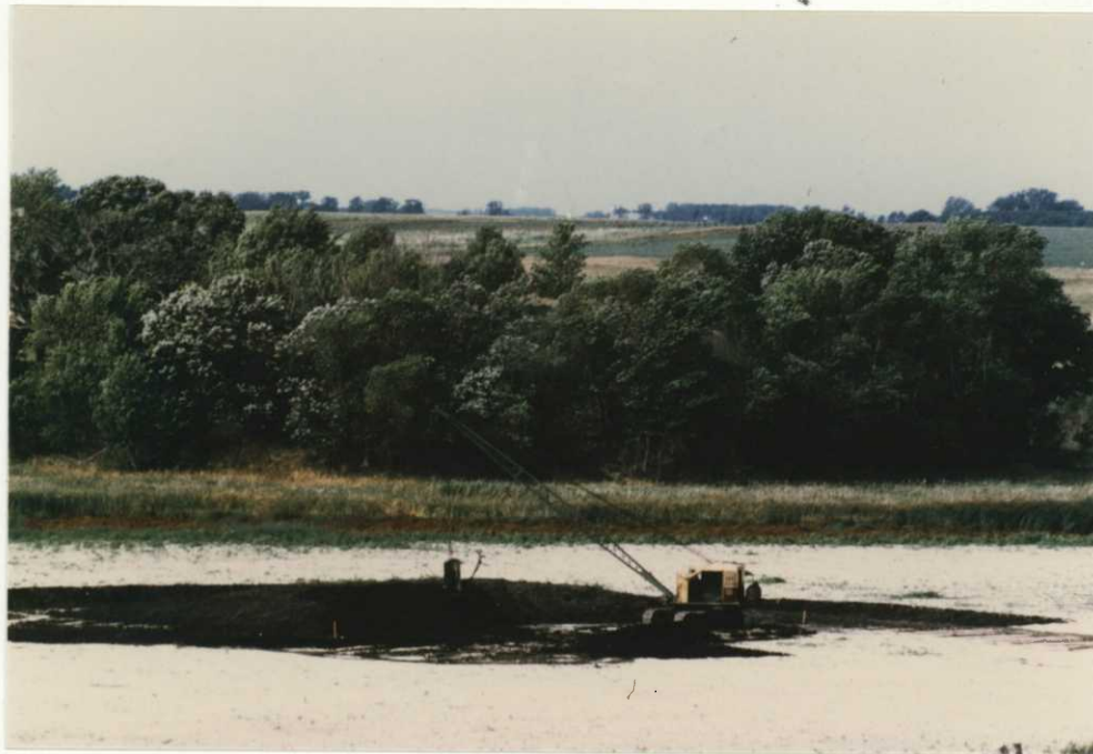
Contractor constructing island in Pool H. 8/3/88 BLA 88-34
