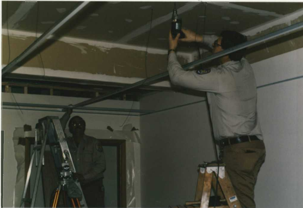
Rodney Ahrndt and Victor Gades installing drop ceiling in new basement office space. 12/31/88 BLA 88-39
