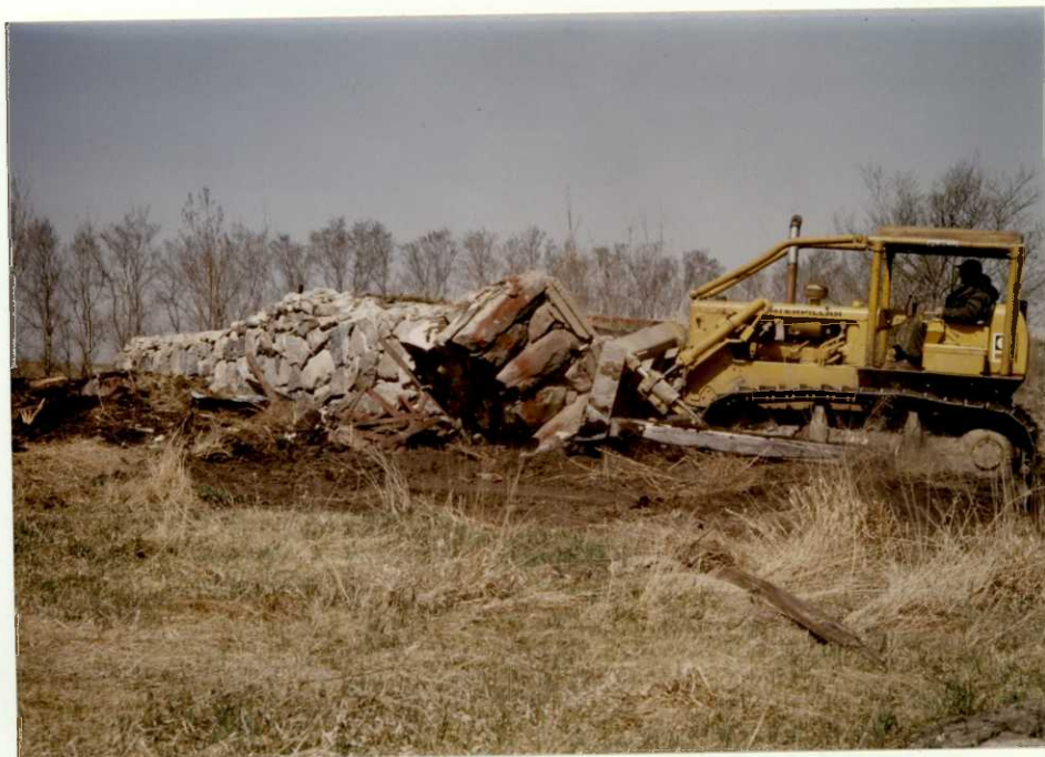
Burying barn foundation on the Larson WPA, Pope County. 81-23 RDS
