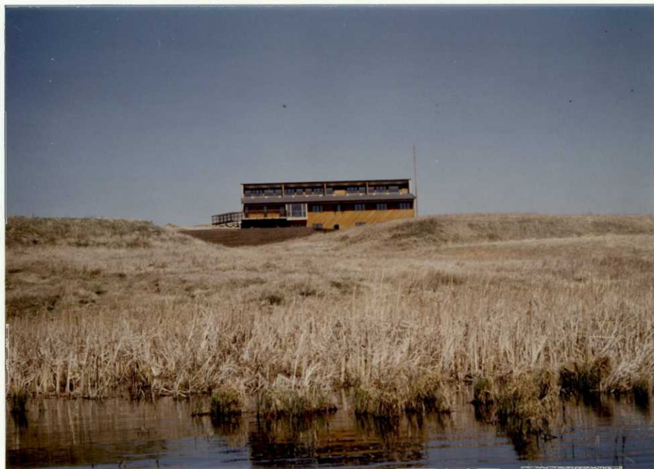
Looking north at the south side of the new office.
