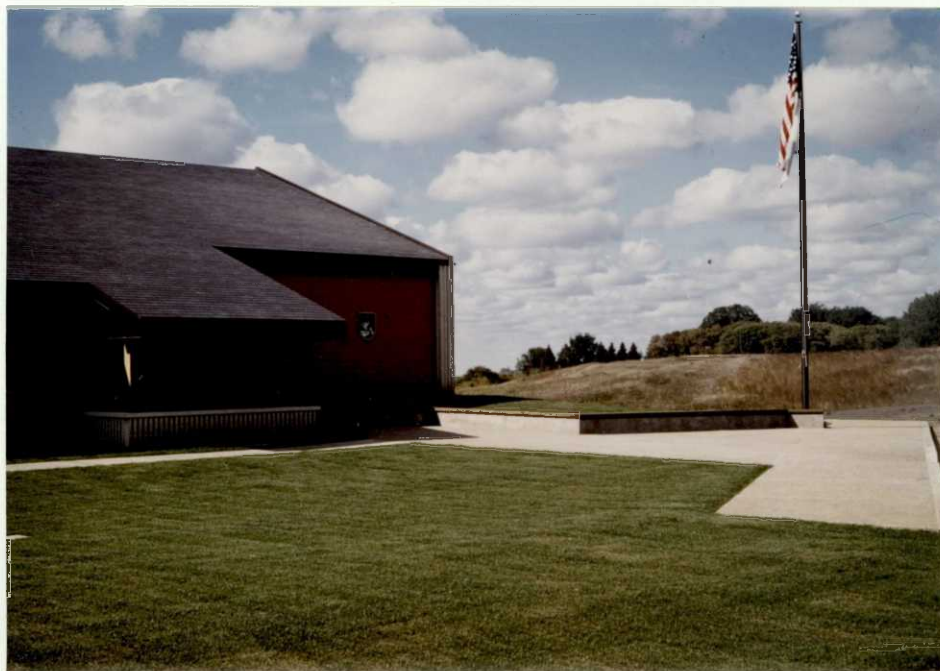
Main door to the office building. 81-20 BLA
