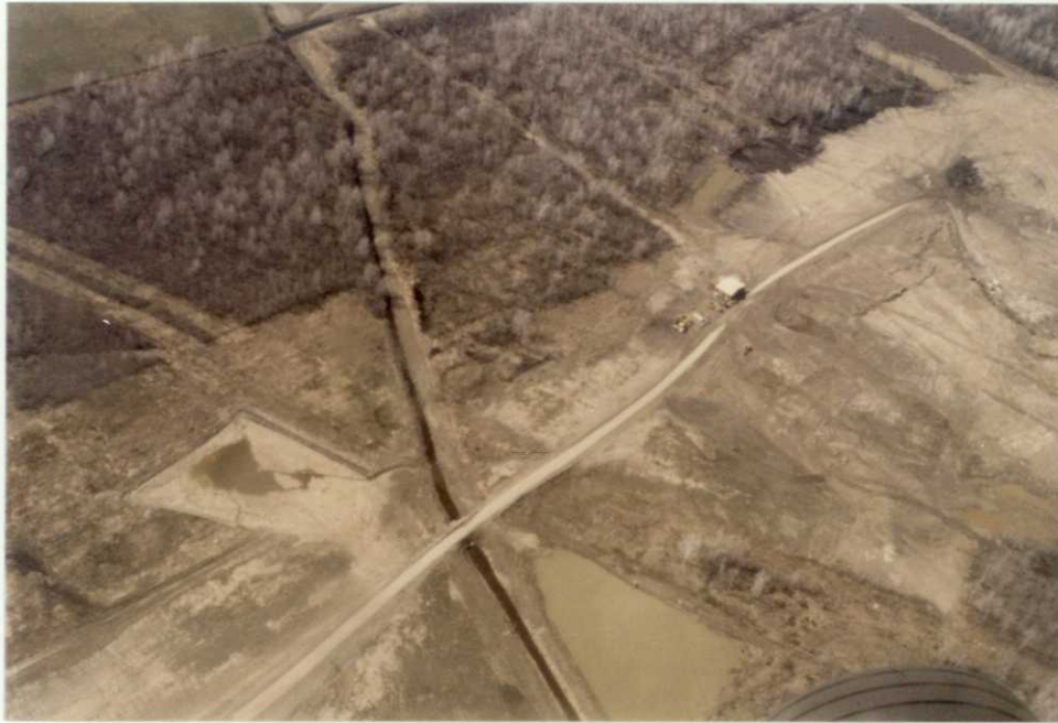
Aerial view showing portion of Tantalito Landfill. Road runs north and south. Note Black Brook bisecting area NW to SE. Also note pooled water around edges of working faces; almost all of these pools are contaminated with leachate. Several heavy metals and some organics have been identified. Photo by Hegge.
