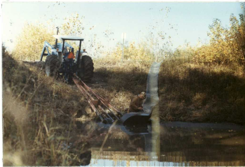
Using diesel Ford tractor with 16" Crisafulli pump reduced fuel consumption by 50 percent compared to operation of Waukesha power unit. (R-970, P-17, TSS) (10-29-84)
