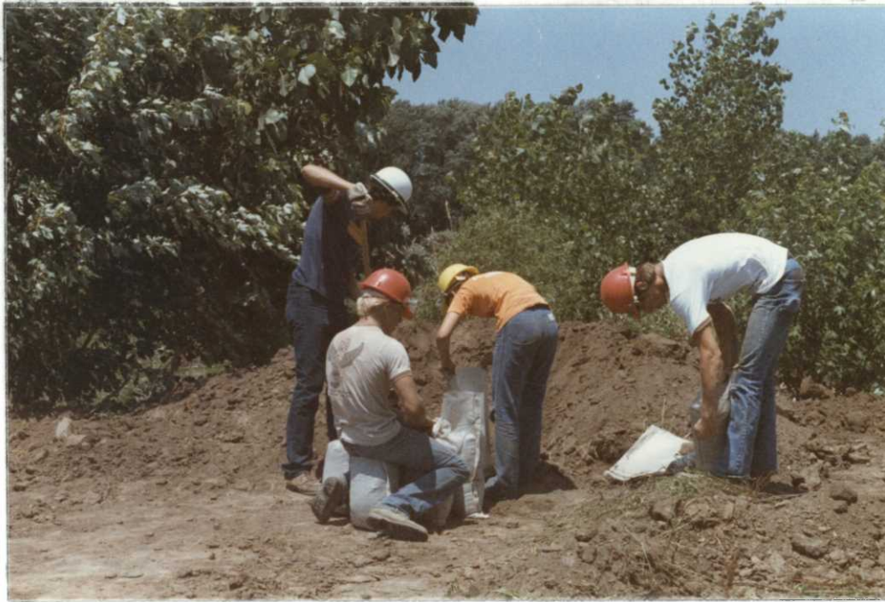
YCC crew filling sandbags supplied by Corps of Engineers. (R-967, P-16, TSS) (06-28-84)
