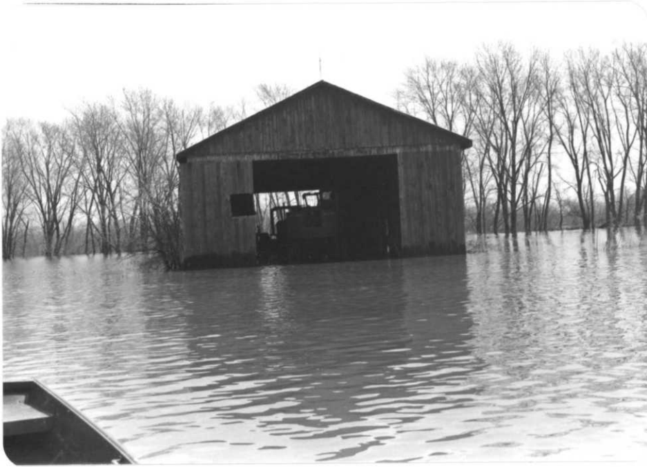
Flooded storage building located on the highest ground. (R-926, P-9, CWW) (4-3-79)
