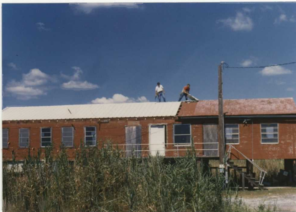
FIG. 9. REHABILITATION OF THE REFUGE HEADQUARTERS BEGINS. (JK)
