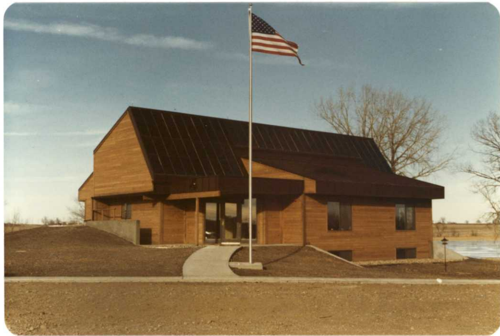
Figure 4. The new solar heated office was occupied in August 1980. 81/1-14 1/23/81 BTS
