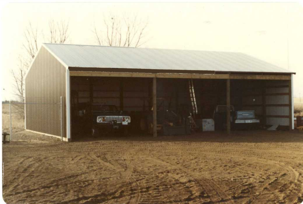
Figure 6. This 36' x 48' pole shed was built force account for additional storage space.
