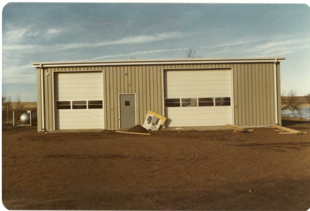
Figure 5. This new shop, a Christmas present for the Biological Technician who has used inadequate facilities for 11 years, will be ready for use early in 1981.
