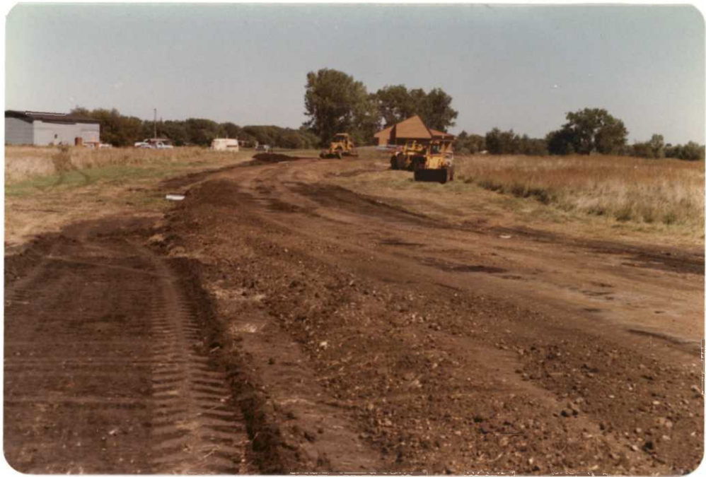
Figure 10. Local contractors (Reinicke) construct the entry road into our new office.
