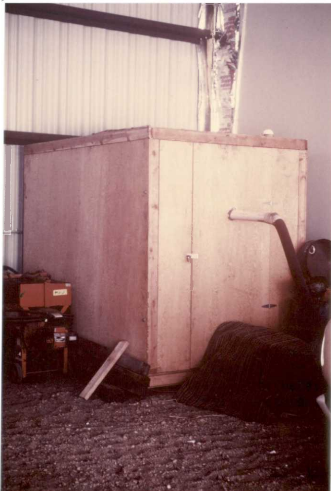
Photo #7 The seed storage facility constructed for native grass seed. The interior has three inches of foam insulation. KAS Feb 1983
