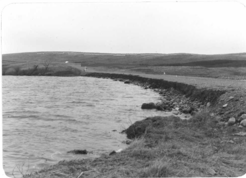
Iverson Dike was raised three feet and widened in October 1975. With the absence of riprap, high water again in April 1976 began eroding the dike's north slope. May 1976
