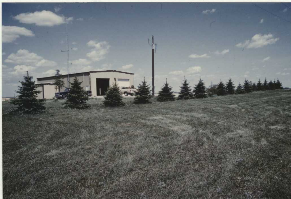
Photo 13. Regional tree spade was utilized to plant this conifer screen planting at our shop site. Trees were obtained at no cost, 4/85 - RAH.
