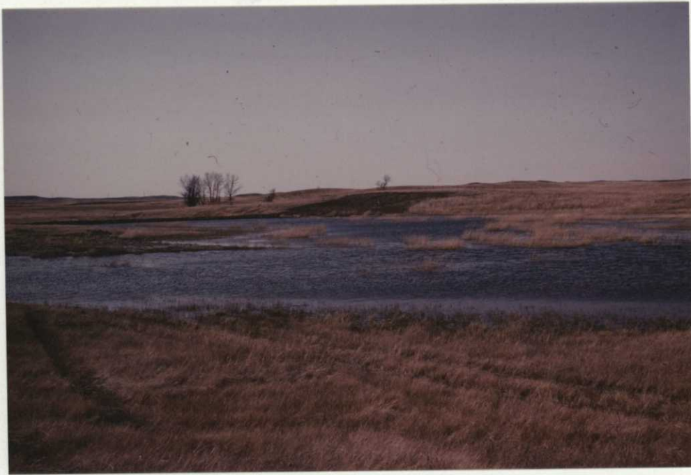
Photo 6. Wetland created after determining proper levels and constructing an earthen dam with overflow culvert, Kautz WPA, 85 - RAH
