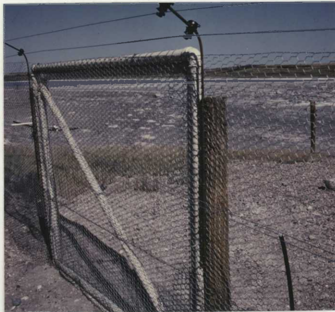
Photo 34. Gate designed into electric fence to facilitate access, West Island WPA, 7/85 - LDW
