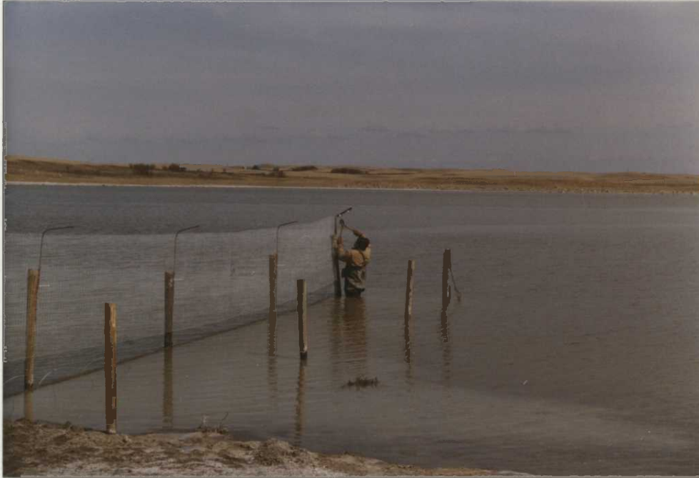
Photo 33. Constructing electric predator barrier fences on into the wetland to prevent predators from simply walking around it, West Island WPA, 4/85 - MG
