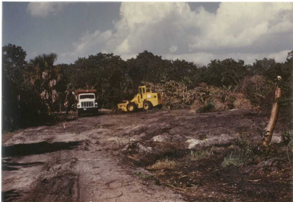
Initial clearing of Maintenance Center site.
