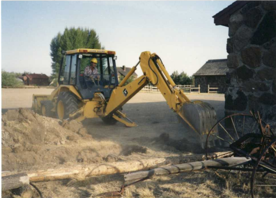
Installation of waterline and faucet for public use.
