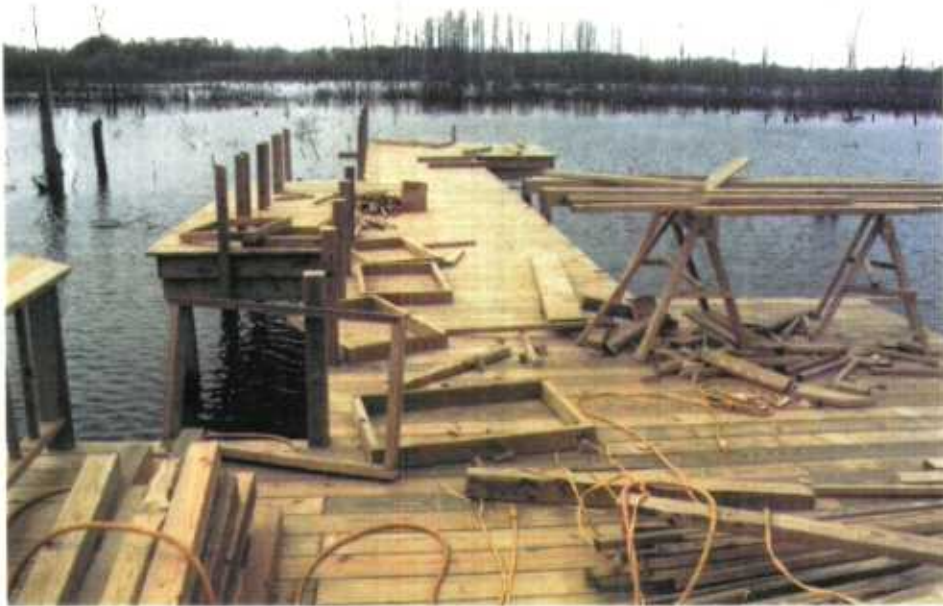
Construction of the first Project Fish facility began October 1992. (R100-04-93, MLN)
