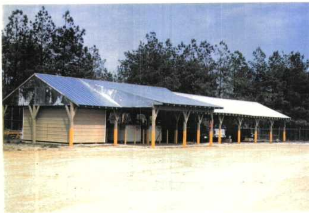
Refuge pole storage shed after rehabilitation. (R200-06-93, GHS)
