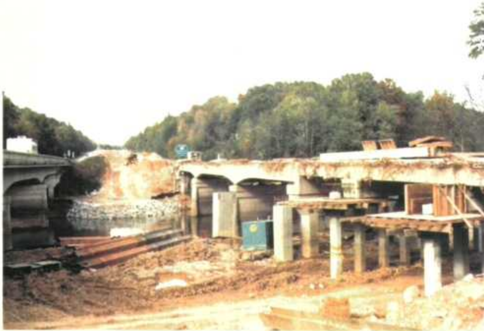
I-40 Bridge Rehab (R200 10-93, GHS)
