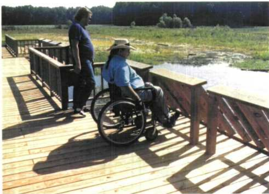
Sloan Lessley, who works for the Arkansas Game and Fish Commission and was the principal designer of this Project Fish facility, makes inspection of the completed structure. The feedback loop from users is a primary part of Project Fish development. (R100-07-93, MLN)
