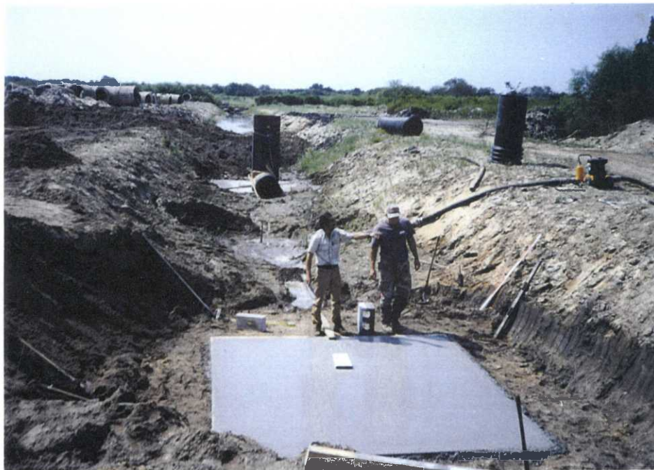
Tractor operator Barrett and forestry technician Gilje complete foundation work prior to the installation of the Goose Pond water-control structure (97-HN4 MJ).
