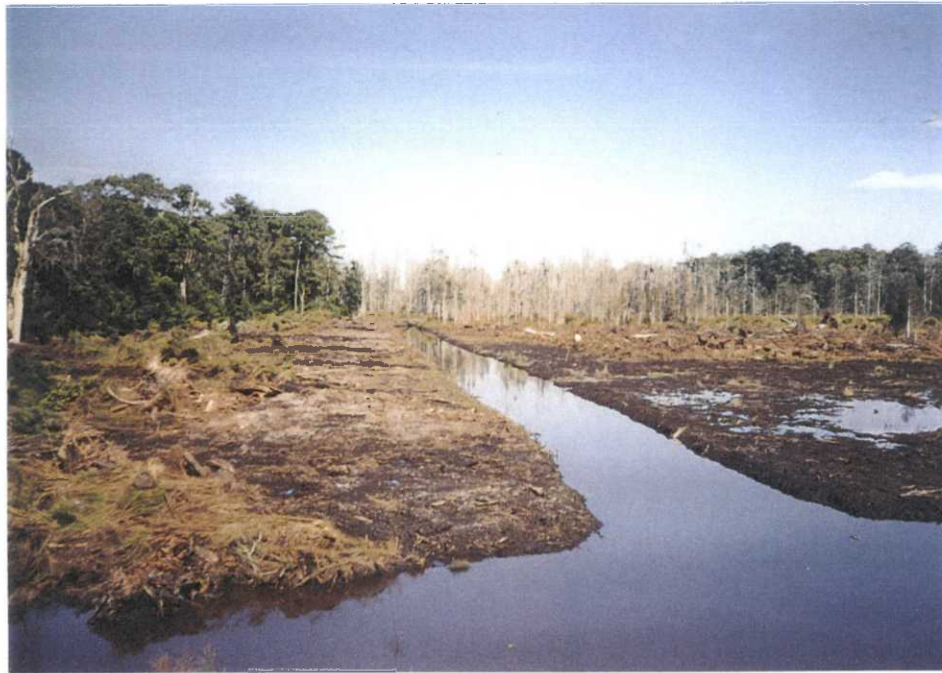
A completed section of the Bluebill impoundment after canal maintenance and root-raking was conducted with an excavator operated from mats (97-HN5 MJ).
