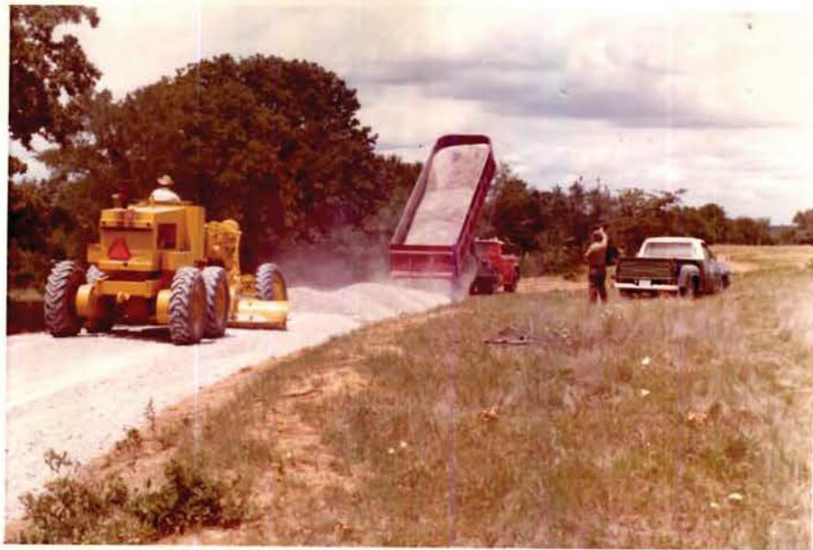
#2 ROAD BASE BEING SPREAD ON ACCESS ROAD TO SANDY PICNIC AREA.
