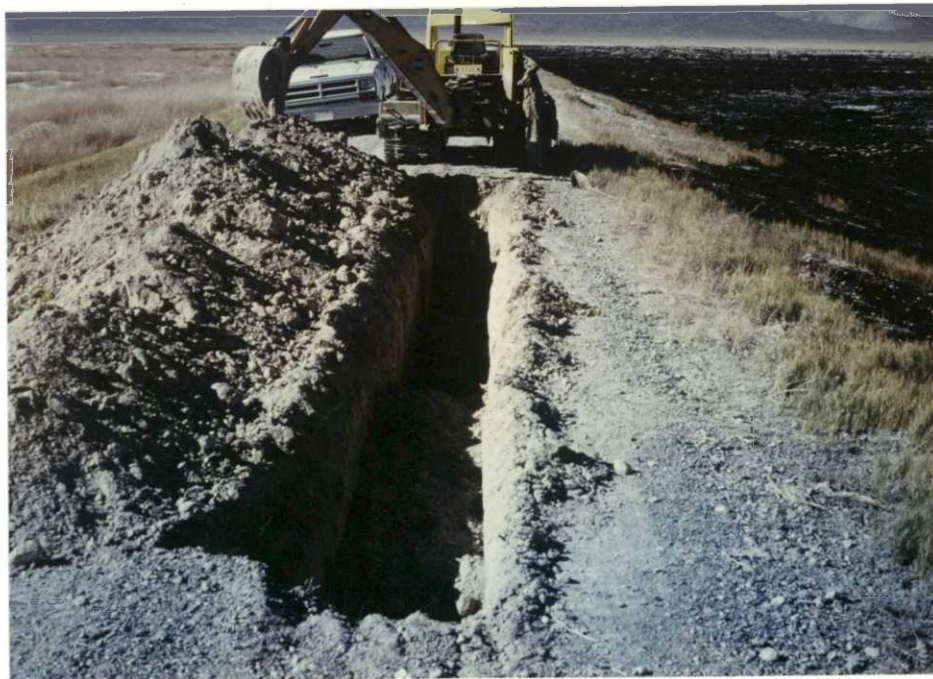
Corrective measures included refilling and packing the dike
