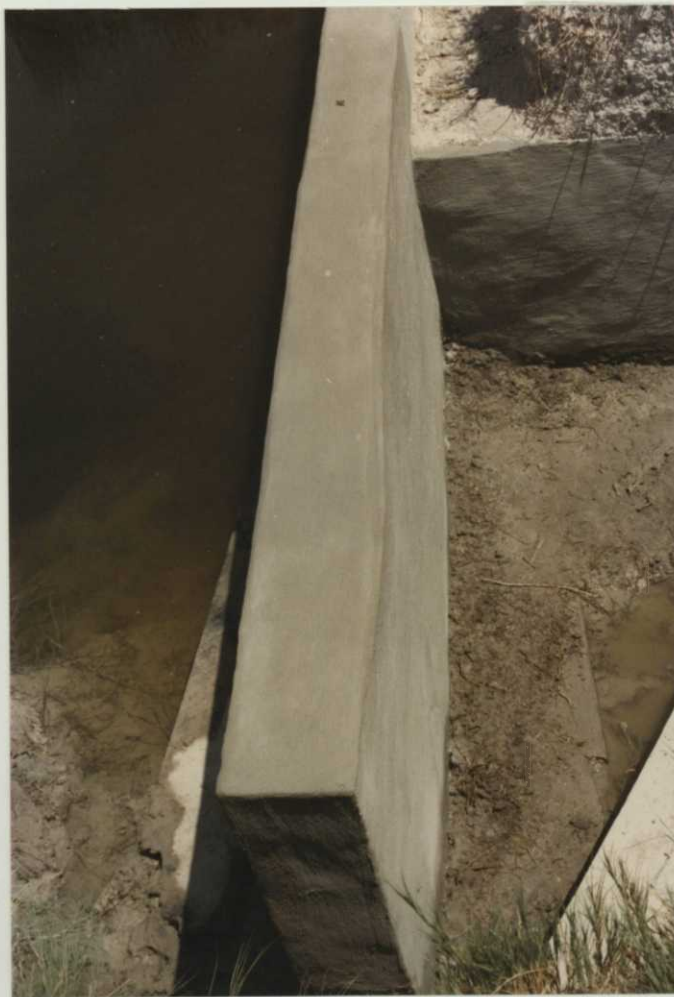
Fig. 8. 7/18/85 North wall (downstream) water control structure #11 after repair. CRD
