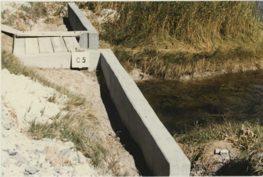
Fig. 15. 9/20/85 WCS C-5 after rebuilding with Thorite. CRD
