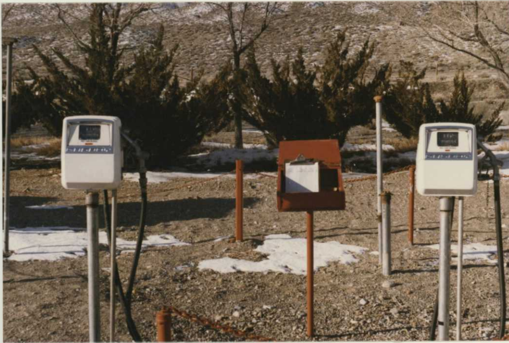
Fig. 17. 1/8/86 A leaky underground tank and two worn-out pumps were replaced. CRD
