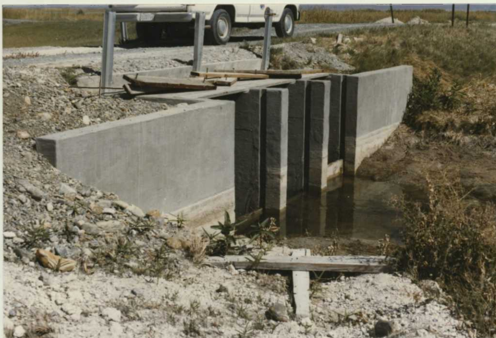
Fig. 11. 9/29/85 WCS #12 after repairs with Thorite compound. CRD
