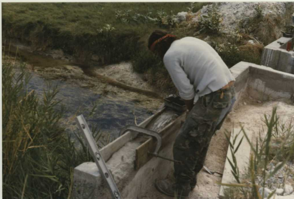
Fig. 13. 8/26/85 Bret Layland uses temporary forms on C-5 for deep fills. CRD
