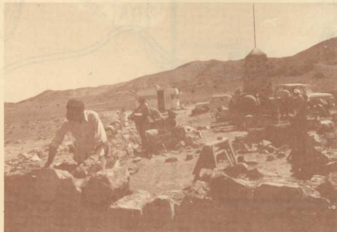
SIMPSON SPRINGS — station site restoration work begins. (1974)
