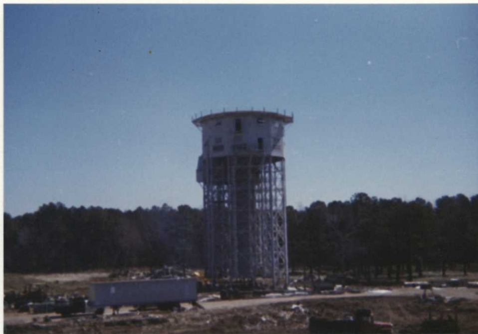
This tower was cut at its base and...
