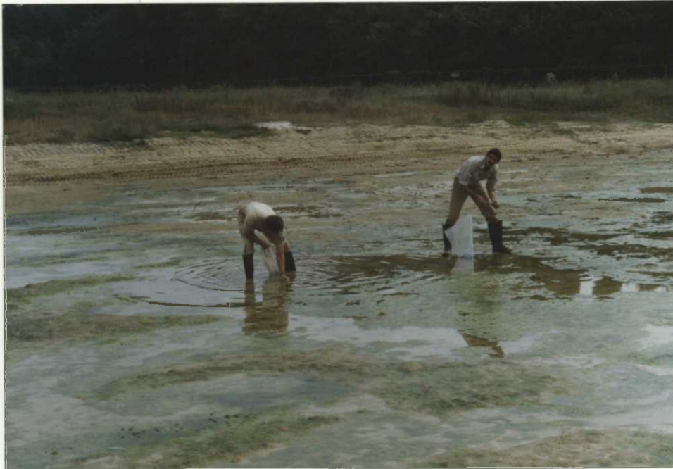
Emergents were planted in the newly developed south pond.
