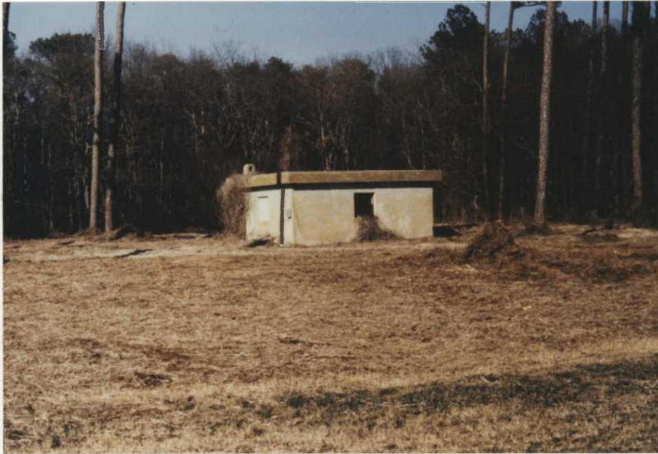
An abandoned Army building from the WWII Fort John Custis days located on the future site of the new office was razed and removed by a contractor. 2/88 L.H.
