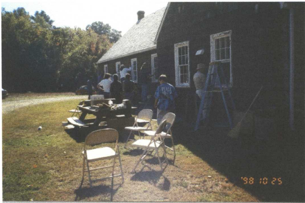
NR-98-21 Scraping and painting lodge windows . . . 10/25/98 MCK
