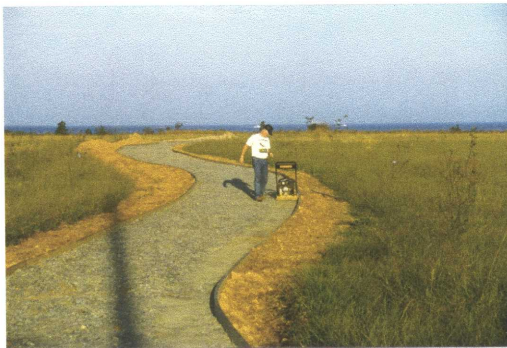
NR-98-16 Watching the tamper do the work!
