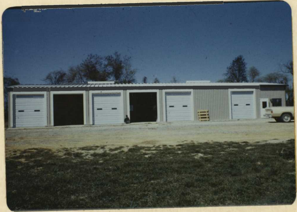
The new metal maintenance building was finally completed in January 1979, courtesy of BLHP.
