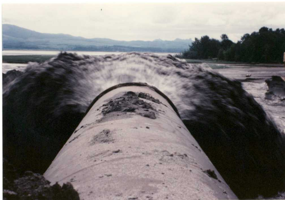
#8-U.S. Army Corps of Engineers conducting a "Beach Nourishment" (dredge spoil) program on Miller Sands Island Spit. The 30" pipe transports 3,000 cu. yds. of material per hour. The dredge operates 24 hours/day, 7 months a year, with a 52-person crew at a cost of $30,000/day. 89-RTV
