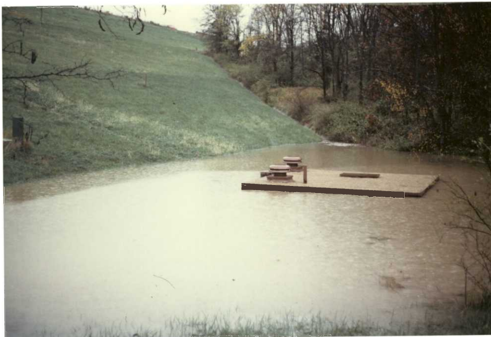
The top of the outlet valve house below Little Grassy Dam. Creek levels rose 15 feet above normal during the November 1 downpour.
