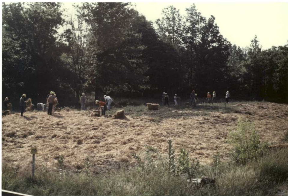
YCC Program accomplishments included seeding and mulching of old building demolition sites. 6/15, 85-6, EFW
