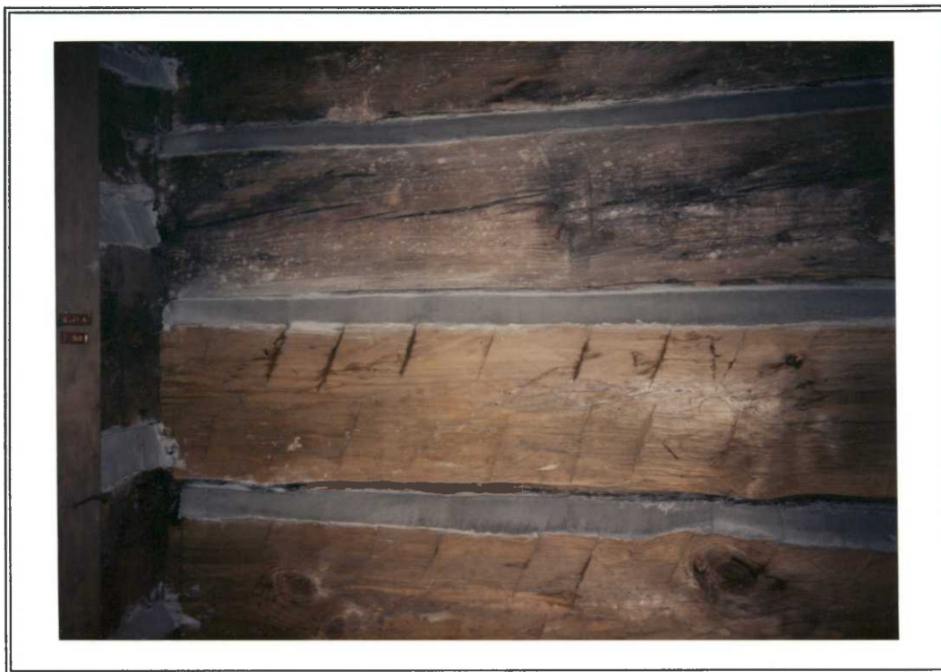
New daubing in place.
