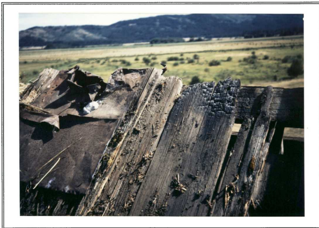
Shakes at peak near old chimney and stovepipe exit. Note charring from past fires. We are lucky to still have a Whitcomb Cabin.
