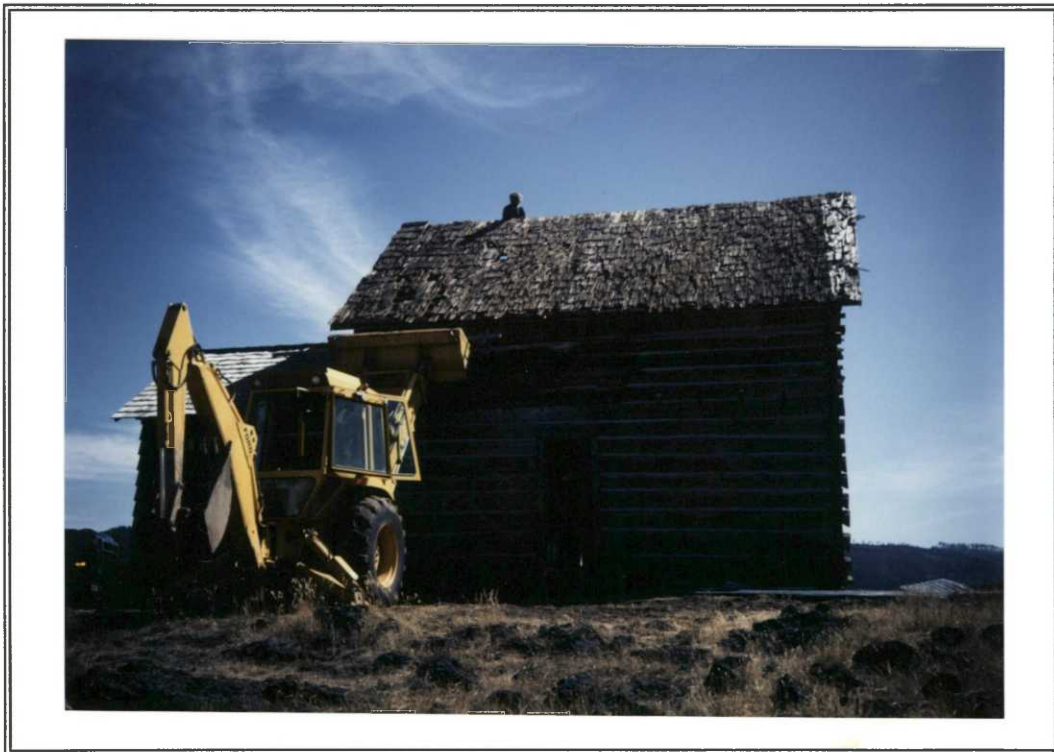
...and is completed. Note metal-covered old shakes on this side.
