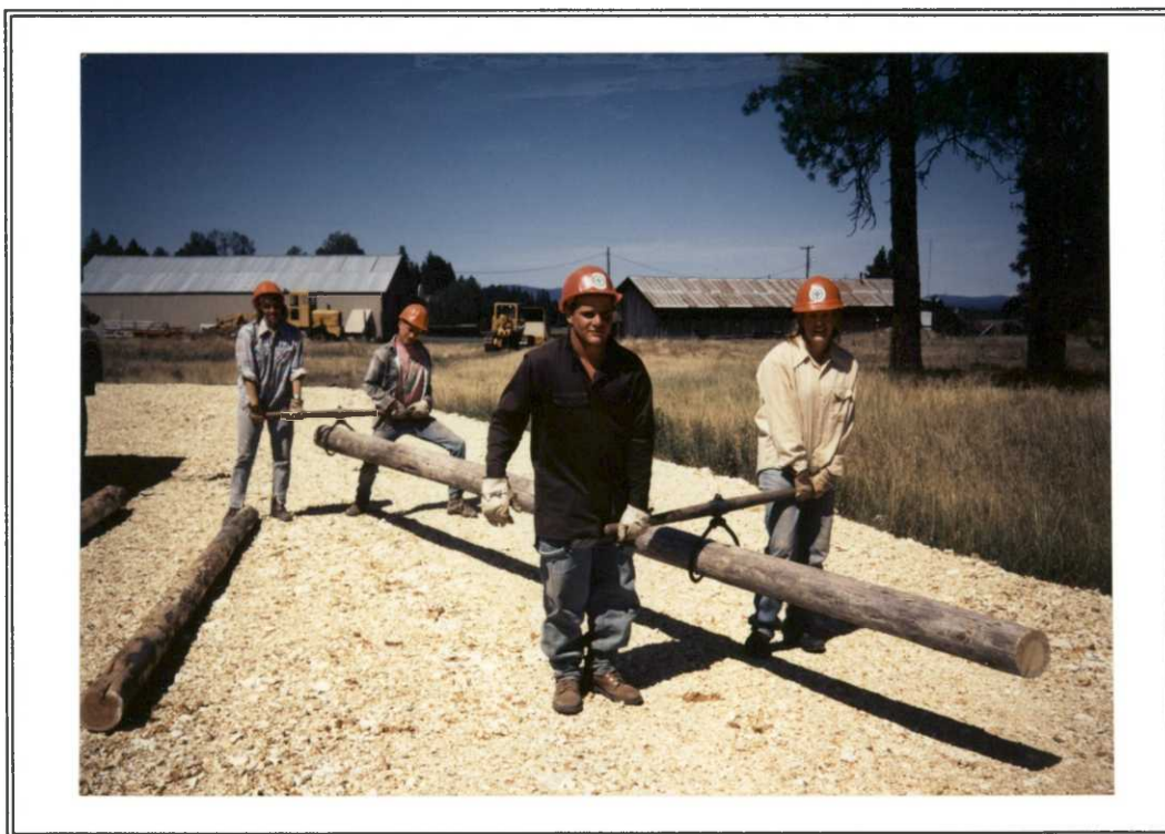
Moving parking bumpers into place in new headquarters parking lot.
