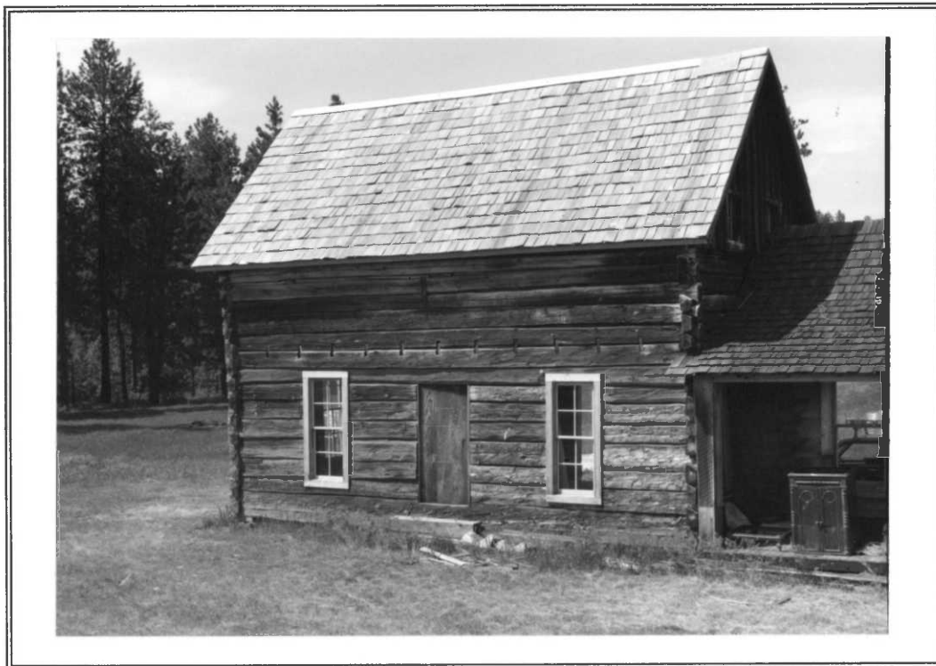
New roof in place.
