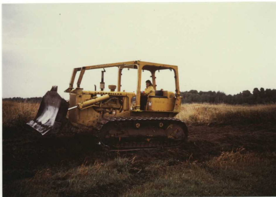
#8-WCC Enrollee Jo Ellen Lively packing section of Camas Ditch bank. 86-HEC
