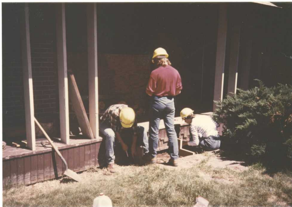
#6-Replacing steps to headquarters residence 84 HEC
