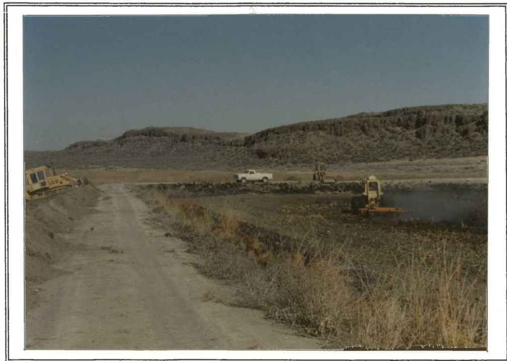
After two years of delays, dikes in Marsh Unit II were finally reshaped and raised, dike tops were graveled, drainage ditches were cleaned, and cattails were disked back. 3/1/90 DEG
