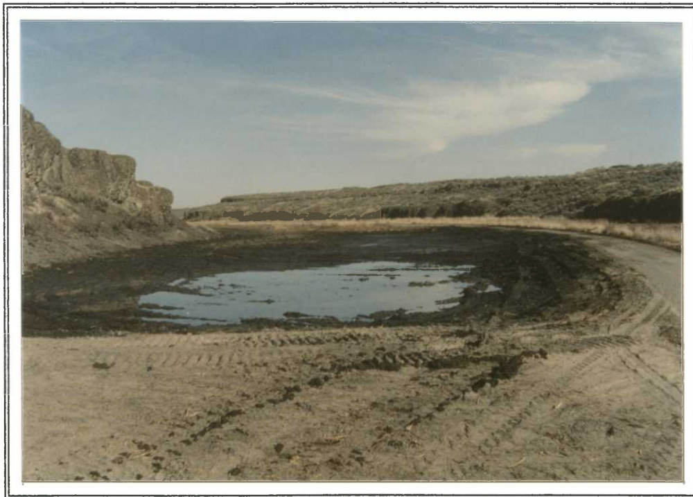
The cleaned impoundments are still too shallow, but significant additional improvements would require a major design overhaul and reconstruction of the entire marsh unit. 3/30/90 DEG
