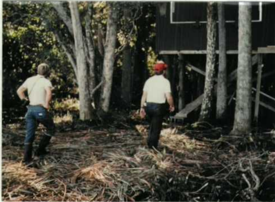
Carl Melberg, Corps, and Charles Bradley, County Health Dept. inspecting fill and septic tank violations. 1983 -3F14 SJM
