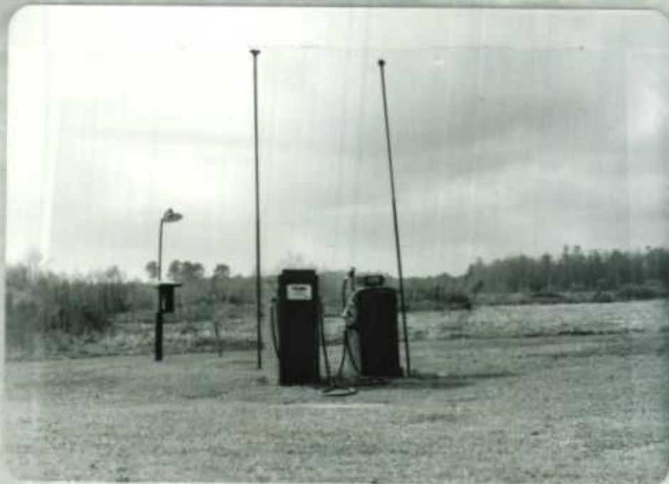
Fuel Dispensing Facility Before BLHP Funds CH-12-78-EC
