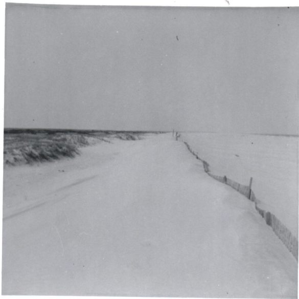
Dune Erosion Control - sand dike and fence - C Dike to wash flats - completed Fall 1956 -
