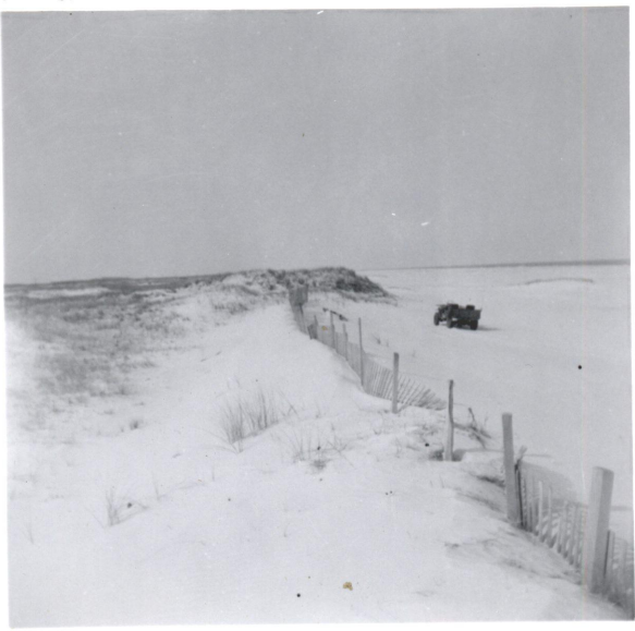
Dune Erosion Control - sand dike closing a break in the dunes - some migration of beach grass - Old Field area -
