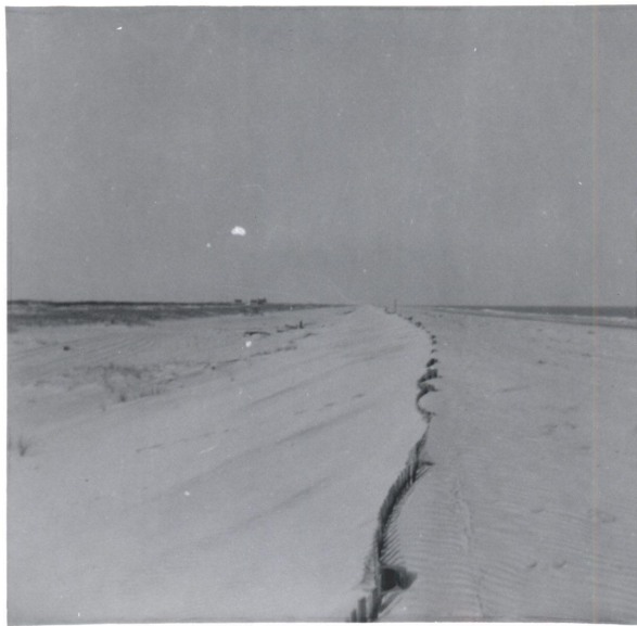
Dune Erosion Control - sand fence and dike - Maryland - Virginia line to Old Field - completed March 1955 - note some migration of beach grass -
