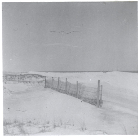
Dune Erosion Control - sand dike closing gap in the dunes - note lack of sand collection - Old Field area -
