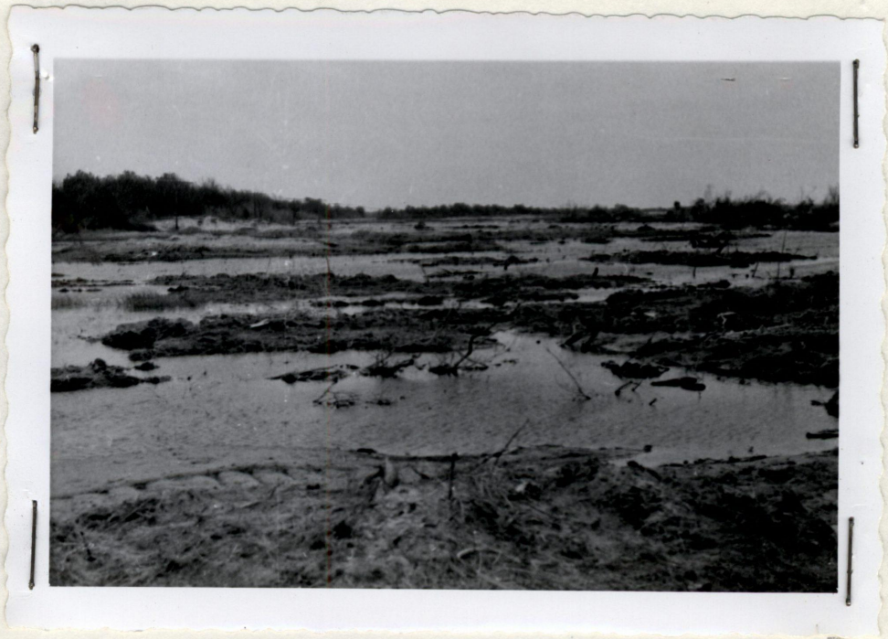
BRUSH CLEARING - AFTER - North of D Dike (refer to p. 4 & 7).
