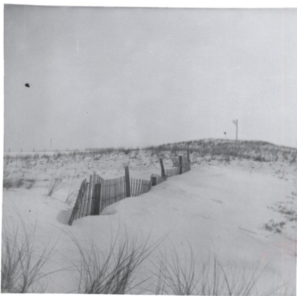
Dune Erosion Control - small sand dike with 50' panel - beach grass moving in -
