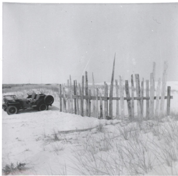
Dune Erosion Control - experimental sand panel made from drift lumber - to close small break in the dunes -
