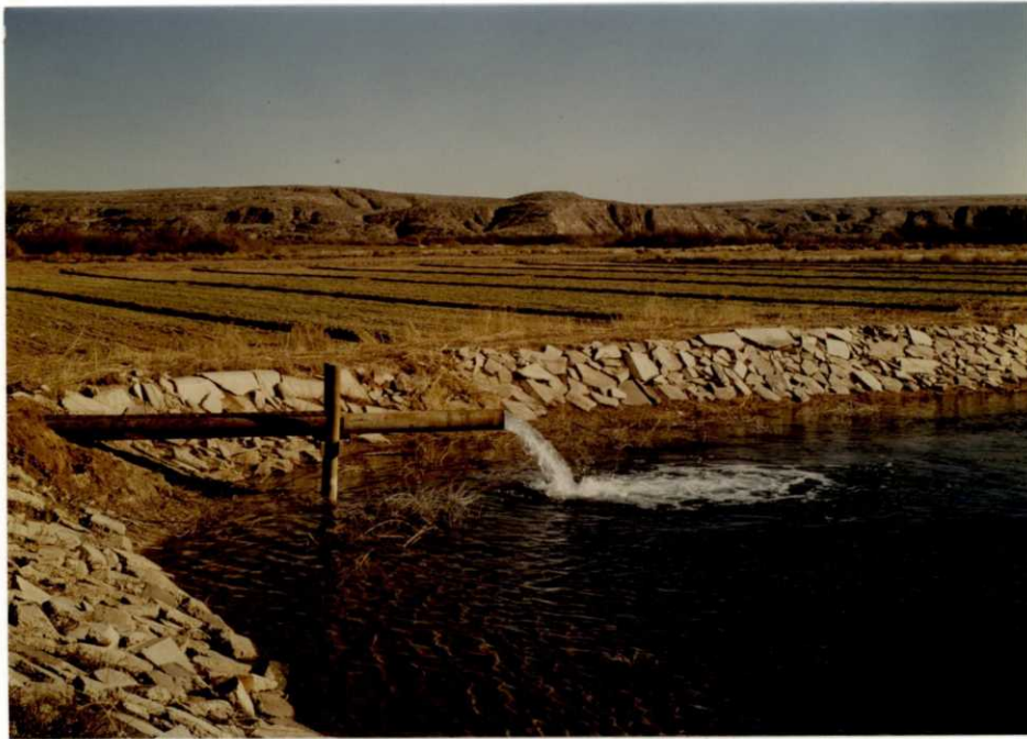
#3 - The irrigation reservoir was rip-rapped with broken pieces of old concrete ditch lining to curb bank erosion. 12/81 LBM
