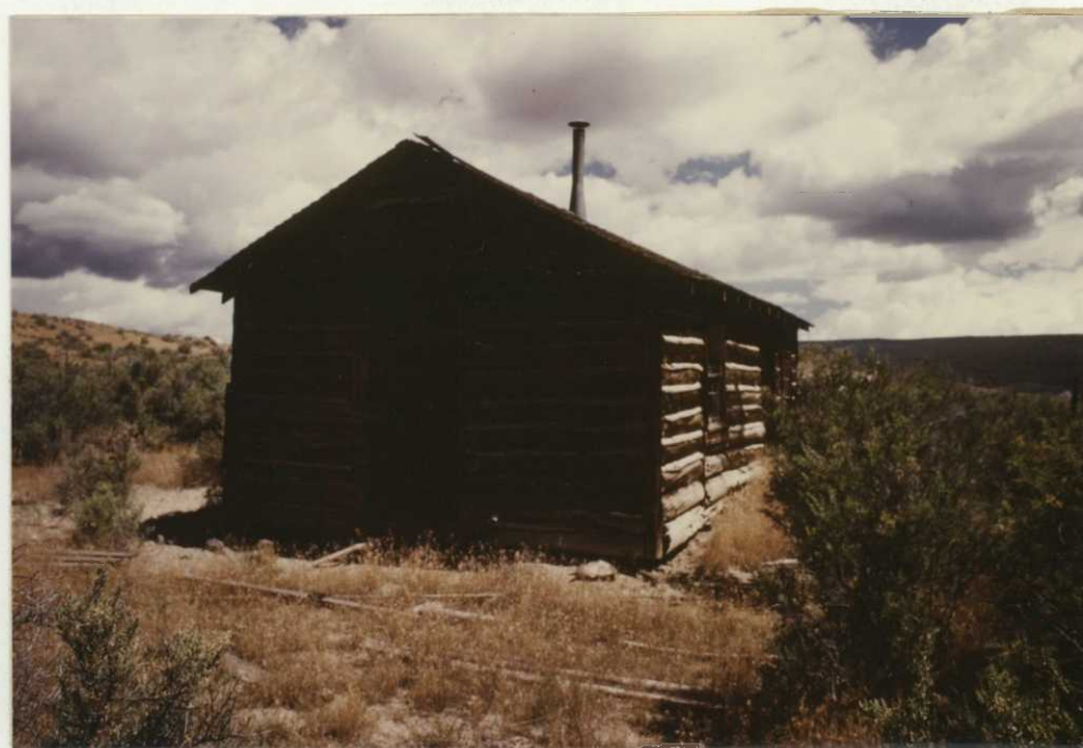
Photo 26. The bunkhouse at the Two-Bar historical site is in better shape than any of the other buildings at the site. 7/24/86-62, JC.
