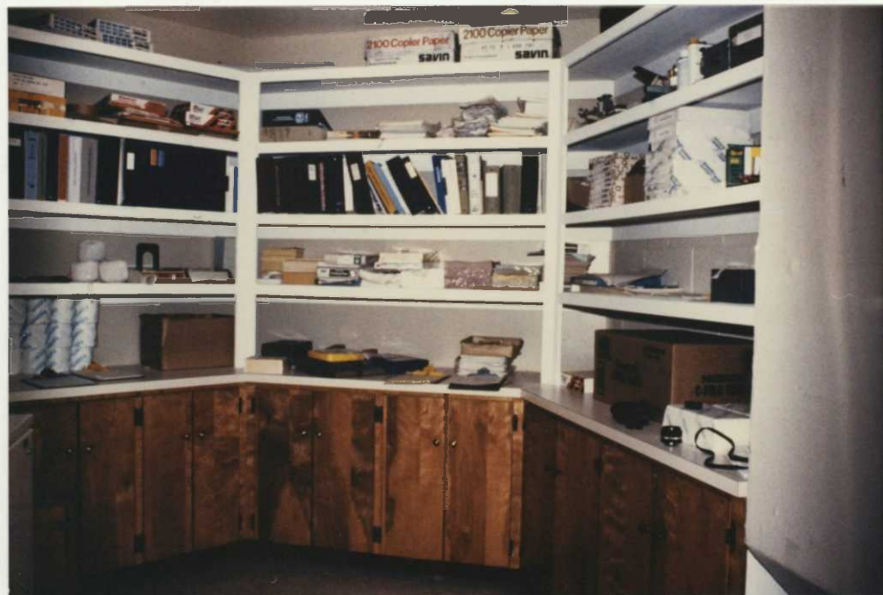
#31 Richard did a fine job on installing a set of new cabinets in storage room #1 of the headquarters building.
