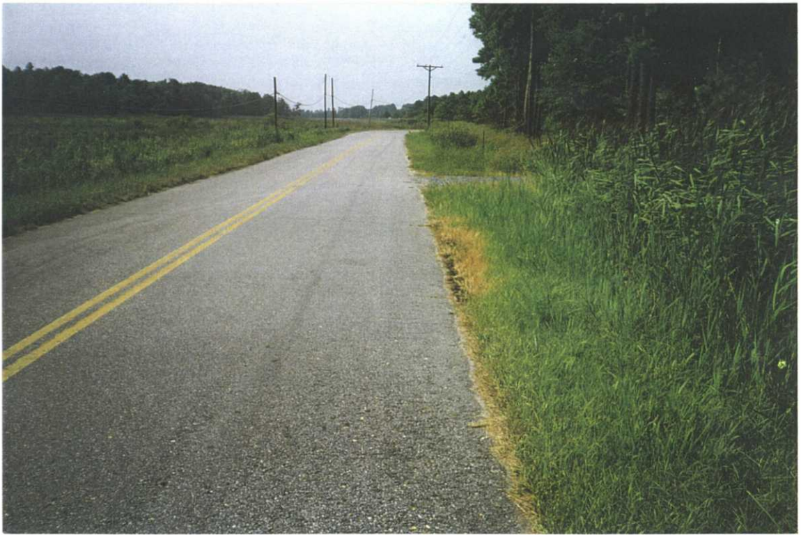
Photo 52. along a four mile stretch of Smithville Road.
