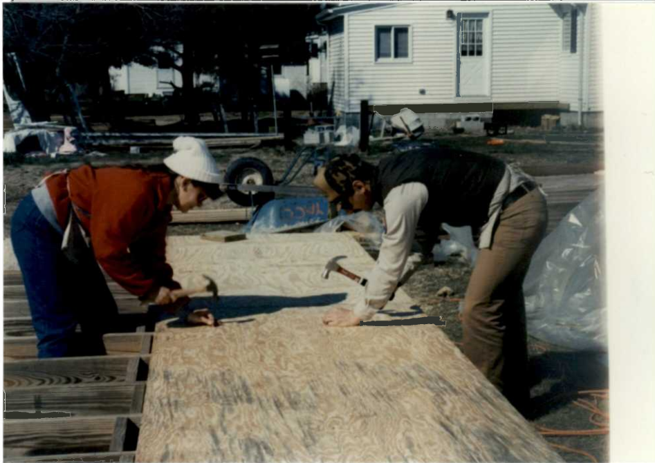
Volunteer Barker and Refuge Operations Specialist Barker working on Martin workshop (photo taken just after air-nailer broke). ROW 3/91
