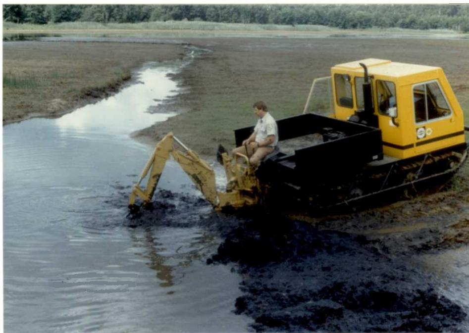
TESTING! TESTING! An attempt to open old drainage ditch in Pool 1 was made in July, using the Bombardier and backhoe attachment; result was helpful but conditions toward the center of the pool were too wet and unstable. LPH 7/91
