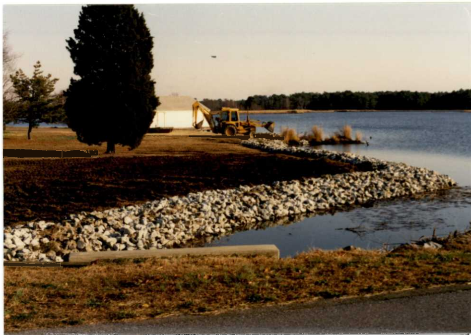
Rip-rap was placed along the Little Blackwater River, south of Quarters 1. GCH 12/91
