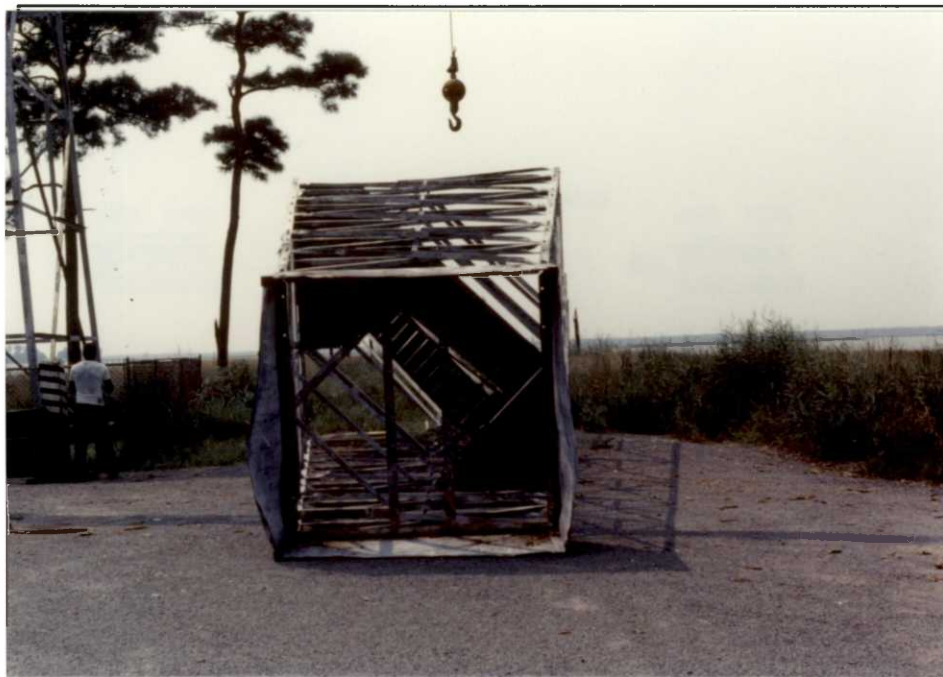
Blackwater's unsafe observation tower was removed. GCH 9/91
