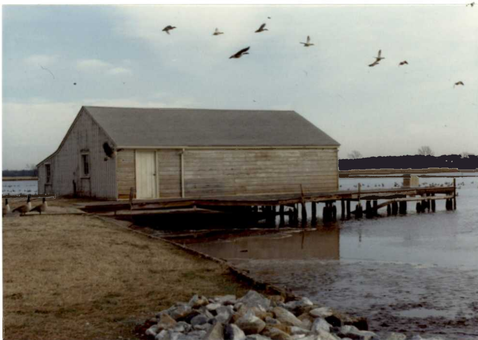
Asbestos shingles were removed from the boathouse, also. GCH 12/91
