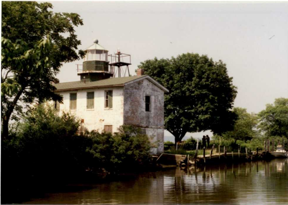
Battery Island and deteriorated lighthouse.
