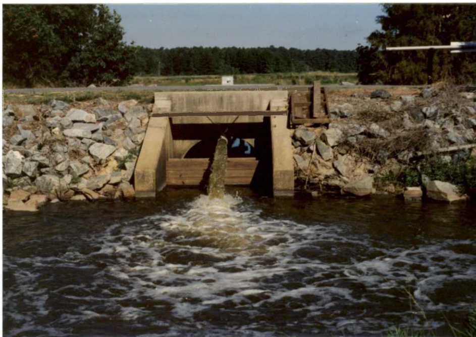
Maintenance pumping in Pool 1 to remove excess water in early June. LPH 6/91
