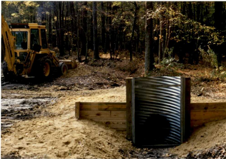
Two water control structures were installed to divert runoff water to Pool 2. GCH 10/91
