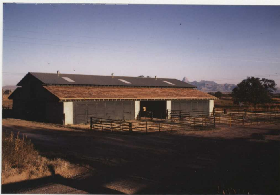
The shake shingle roof was replaced with a new green metal roof with light panels. WAS
