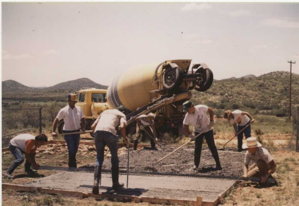
The YCC completing a concrete slab for the San Fernando School as part of a community project. WAS
