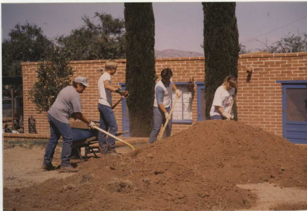
The YCC completed the landscaping of the yard in front of the Manager's residence. WAS
