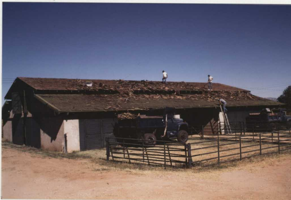
The shake shingle roof was removed from the horse stable by a local contractor. WAS
