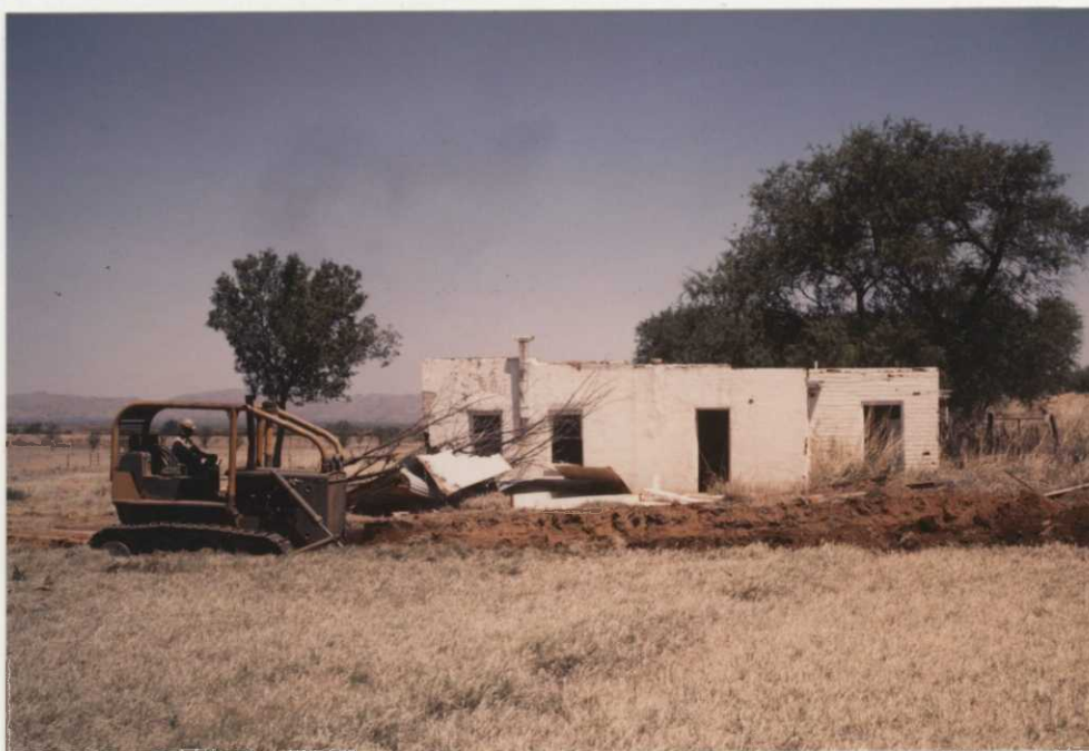
Maintenance worker Dale Enlow in the process of digging a hole to bury an adobe house flooded in 1983. WAS
