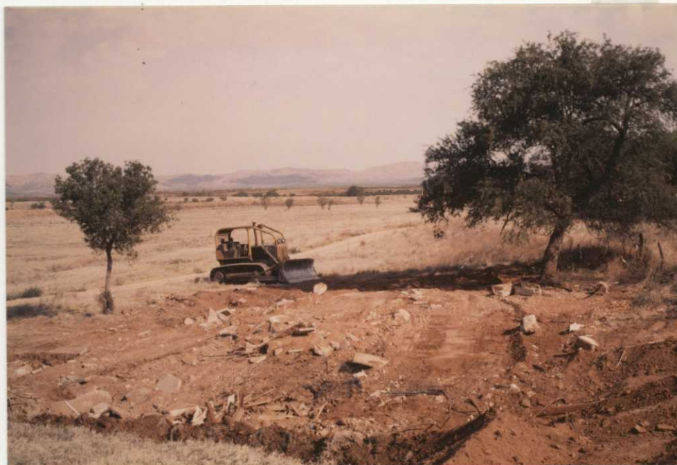
Dale putting the finishing touches on leveling the land after causing the adobe house to disappear. WAS
