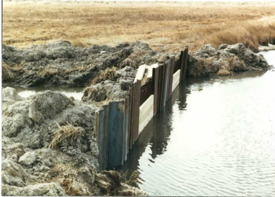
94 NR38 10/27/94 ECP Mortenson Lake outlet control structure.
