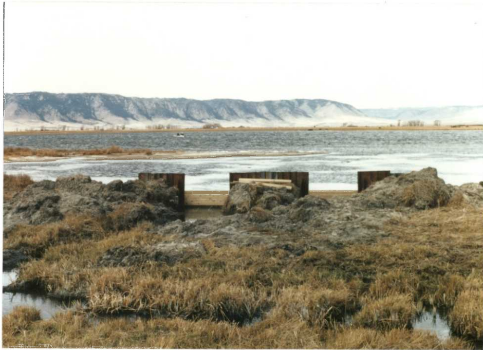
94 NR39 10/27/94 ECP Overlooking Mortenson Lake from the outlet structure.
