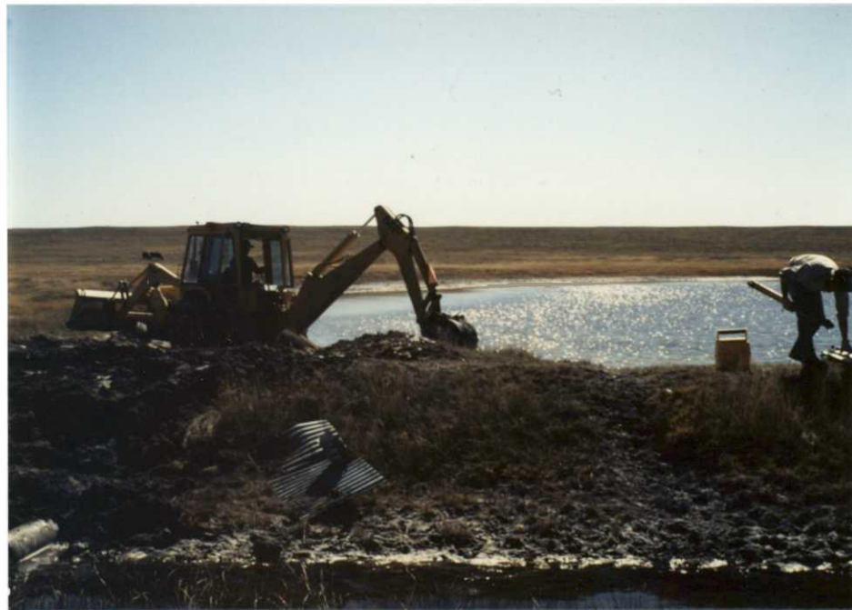
93 NR41 9/29/93 ECP Refuge staff installing outlet at Little Mortenson.
