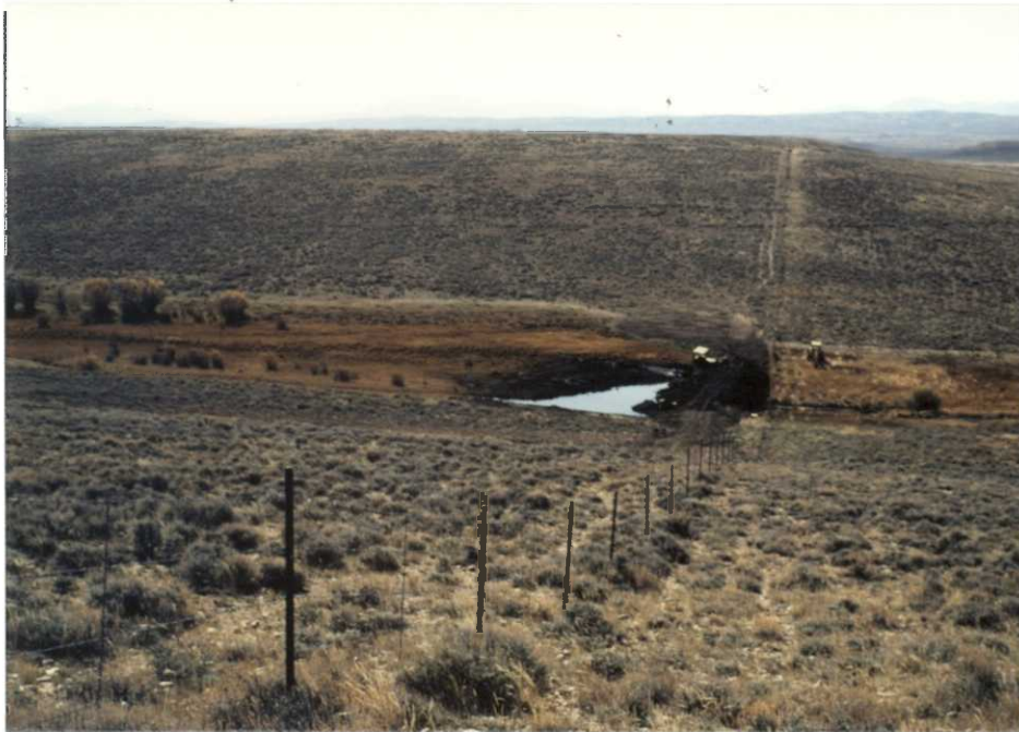
93 NR12 10/6/93 ECP Putting the final touches on Goulette Pond.
