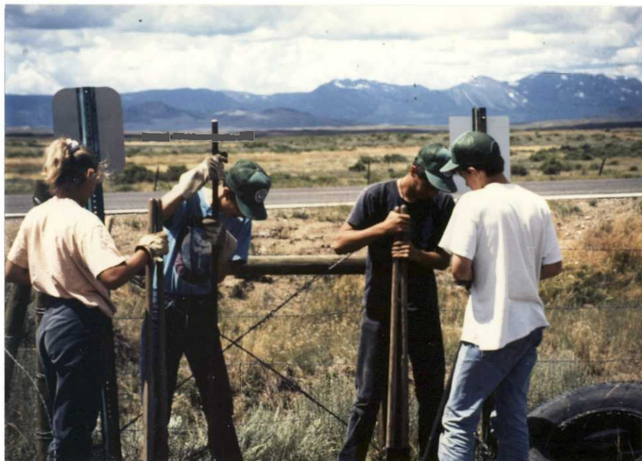
93 NR7 YCC learned the fine art of post hole digging.
