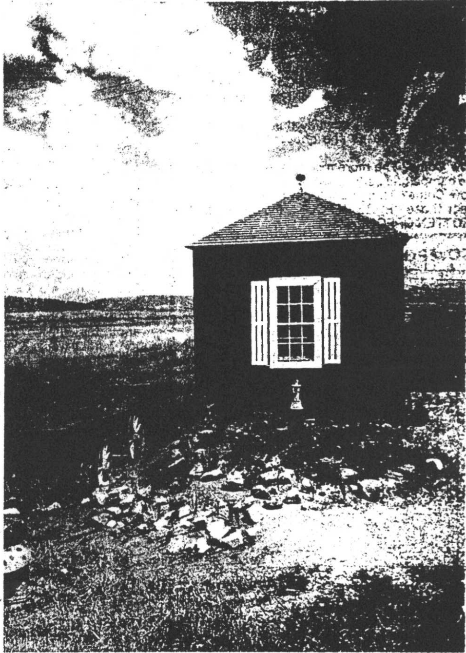
At the north edge of Walden, the redecorated Pump House is a tribute to the efforts of many North Park volunteers this summer. This winning State of Colorado entry in the Make America Beautiful Contest now goes on to regional competition.
