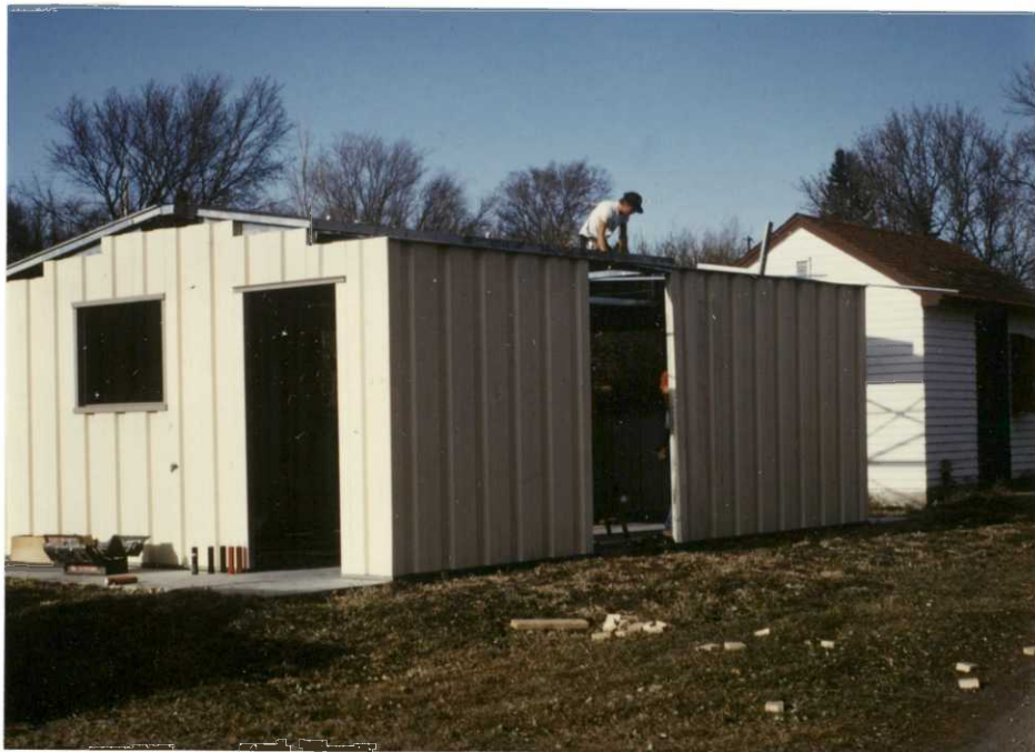
The new oil and paint shed (PVN).
