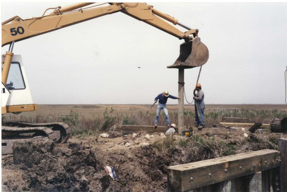
CONTRACTOR INSTALLING NEW BULKHEADS 3" X 10" PILINGS AT COON CREEK STRUCTURE
