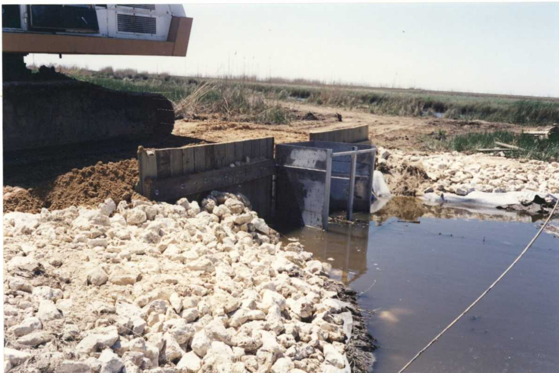
THE GATOR TRAIL ALUMINUM PIPE STRUCTURE NEAR COMPLETION
