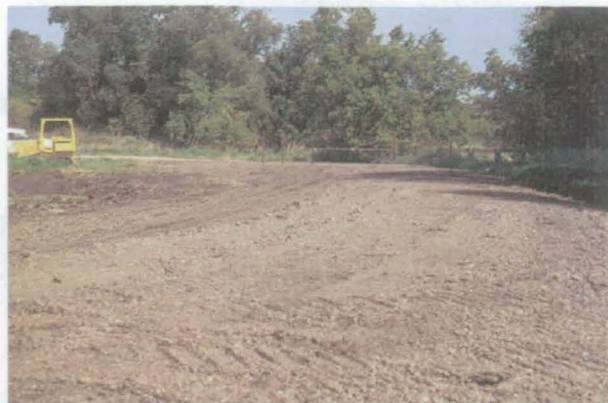
Final Section of Tamarack Dike Rehabilitation Project 8/99 GDT
