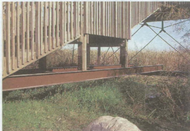
Parker Deck rehabilitation.
